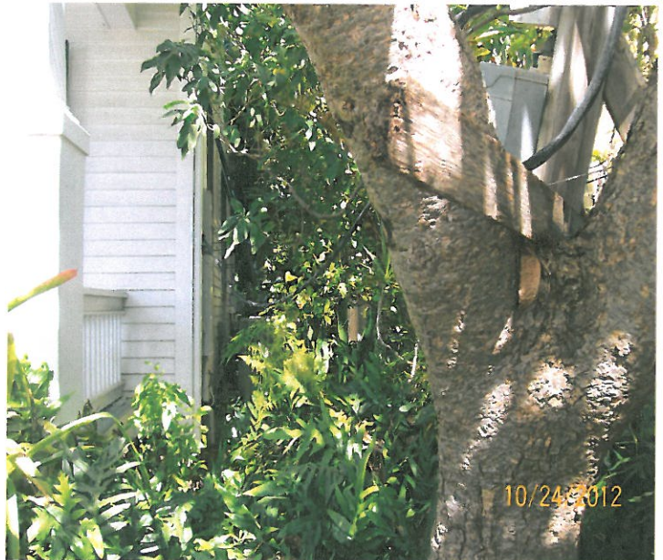
Rear of temporary utility pole. When the pole started to lean against tree—it was braced with a 2x4 nailed into the tree.
