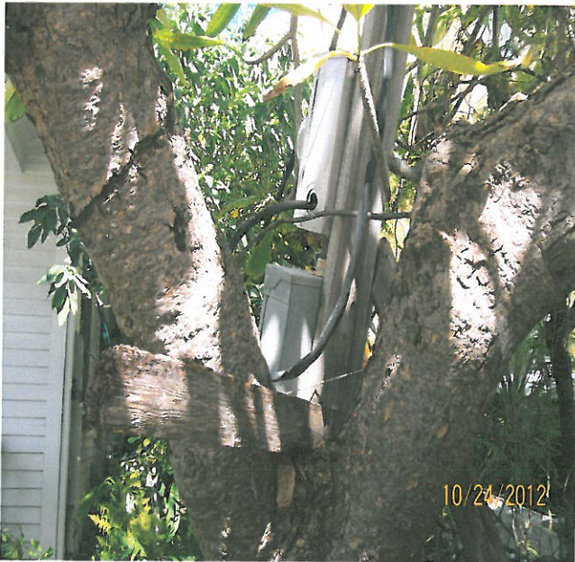
Rear of temporary utility pole. When the pole started to lean against tree—it was braced with a 2x4 nailed into the tree.
