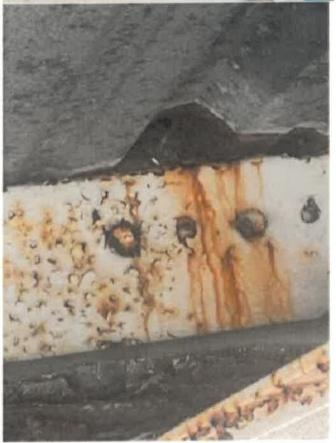
4. light gauge structural columns on the east and western ends of the structure. The cost of replacing these columns is outweighed by the cost involved in cleaning, painting, and ensuring that the existing columns would be up to par, providing the strength required during a high wind event.
