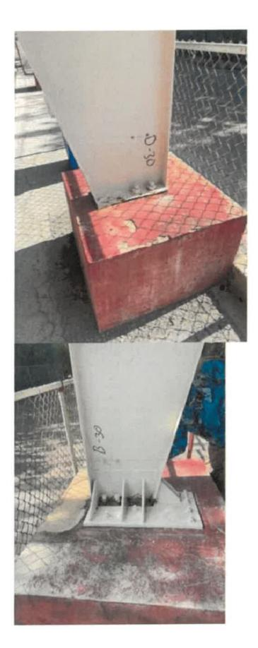
2. Main Bent Structural Bolt Up Plates and Base Plates, after a thorough inspection showed that these joints, for the most part are in good shape, and that the overall condition of the bent is good. The Bents will be cleaned and painted before being reused.
