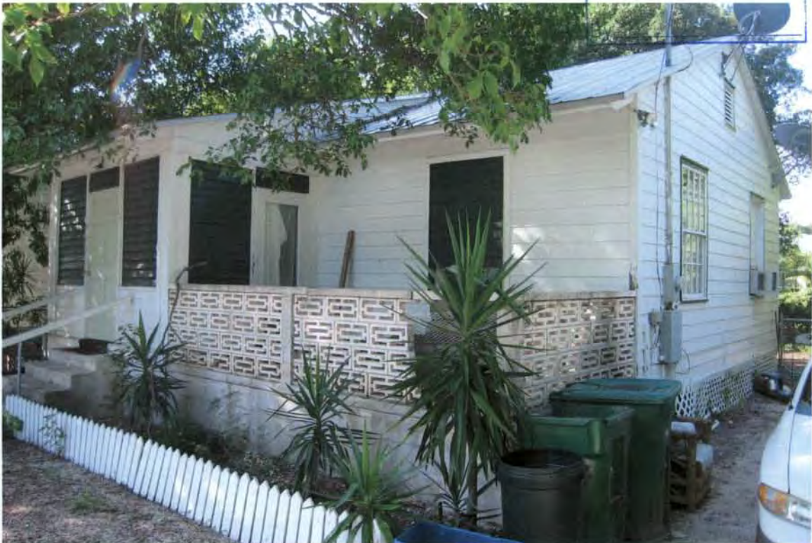
FRONT FACADE OF HOUSE
