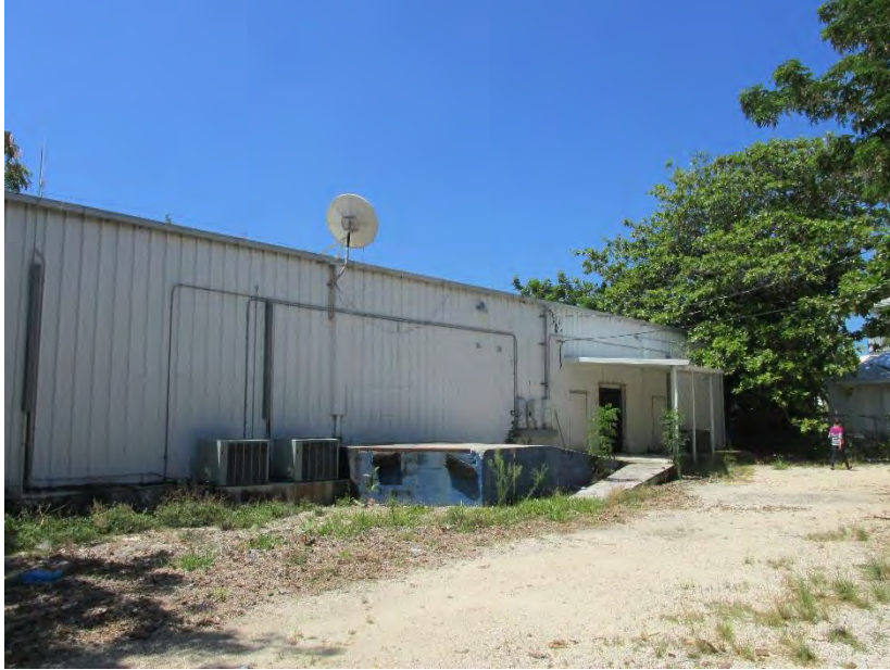
Rear (North) Façade.
