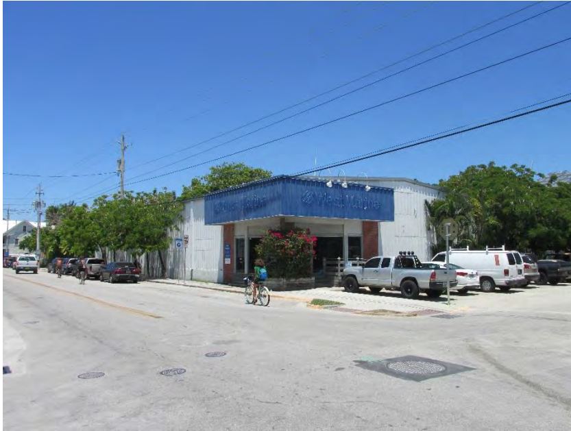
Existing front entry (south and east sides visible). Looking from the corner of Caroline St and William St.
