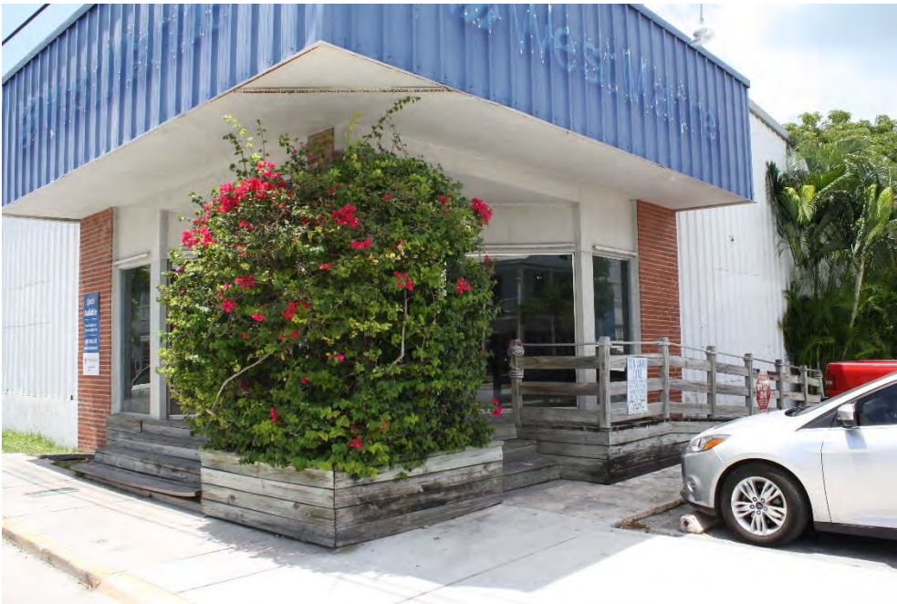
Existing front entry way.
