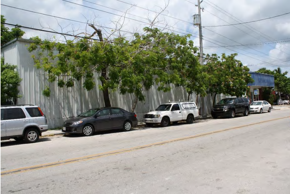
View of South façade. This side faces Caroline Street.
