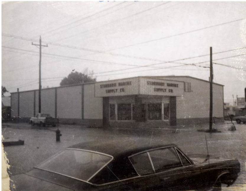
Image circa 1970 of 725 Caroline Street. View of front entry (south and east sides visible). Looking from the corner of Caroline St. and William St.
