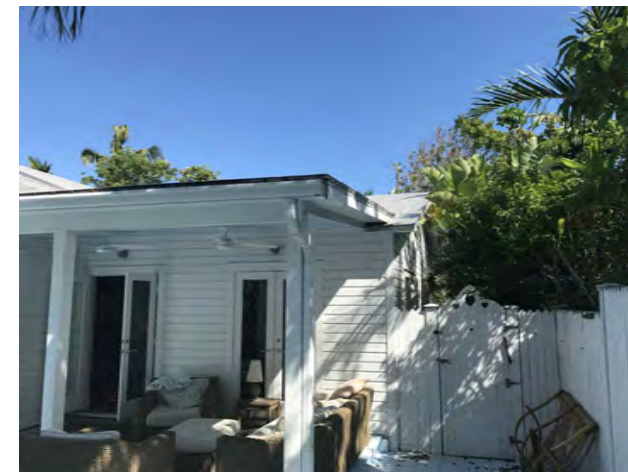
EXISTING S. SIDE OF HOUSE FROM REAR
