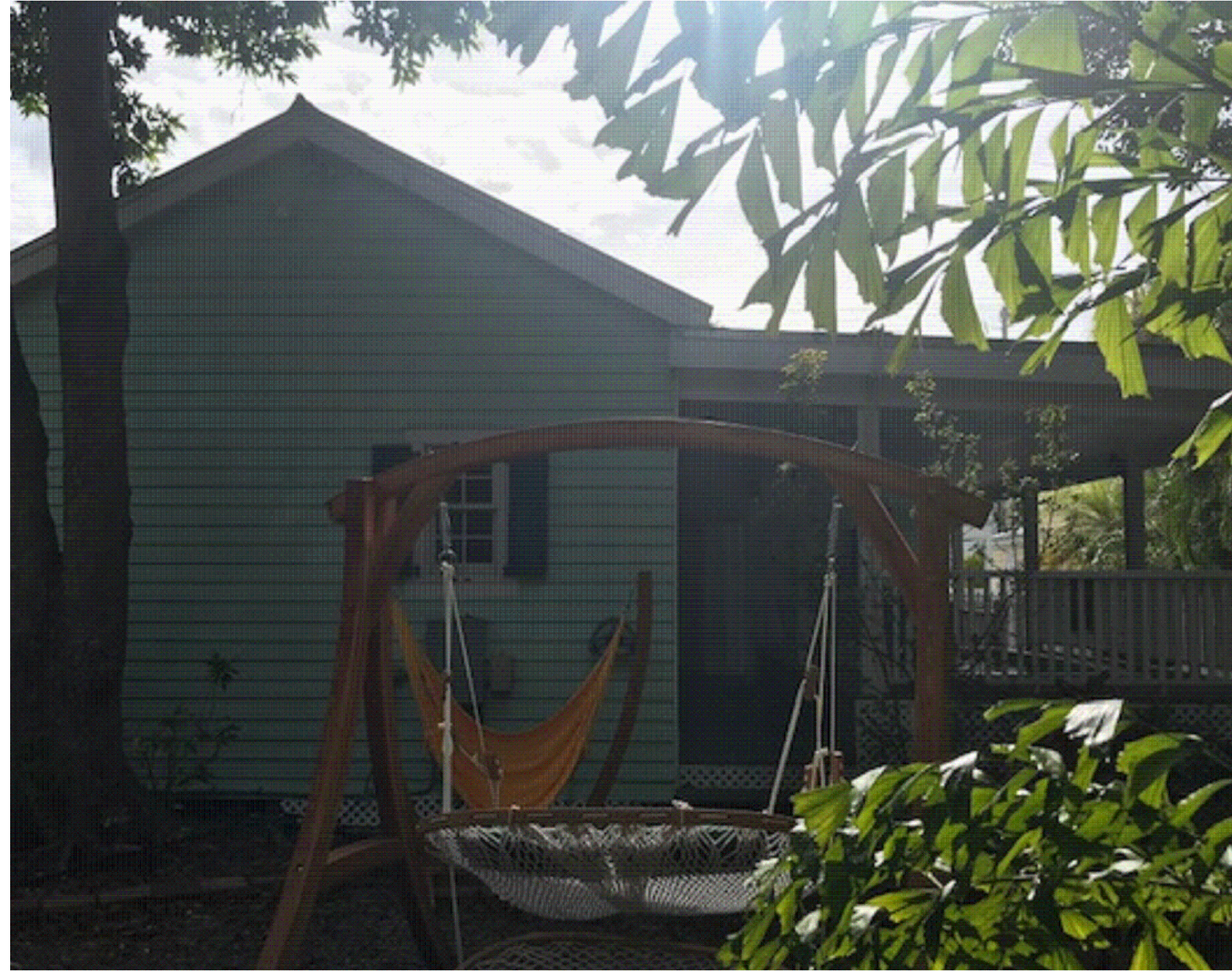
3 PHOTOGRAPH OF EXISTING NORTH ELEVATION
