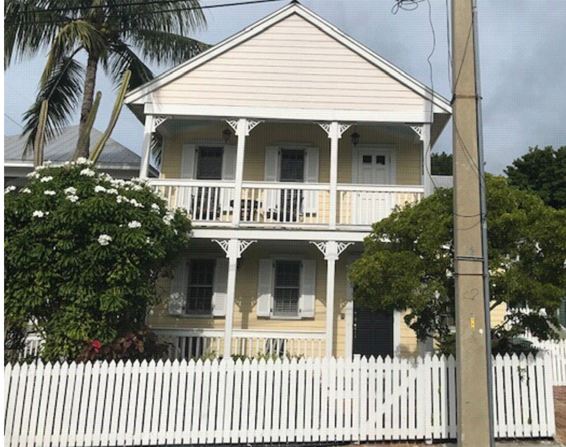
5 PHOTOGRAPH OF ADJACENT PROPERTY TO THE WEST
