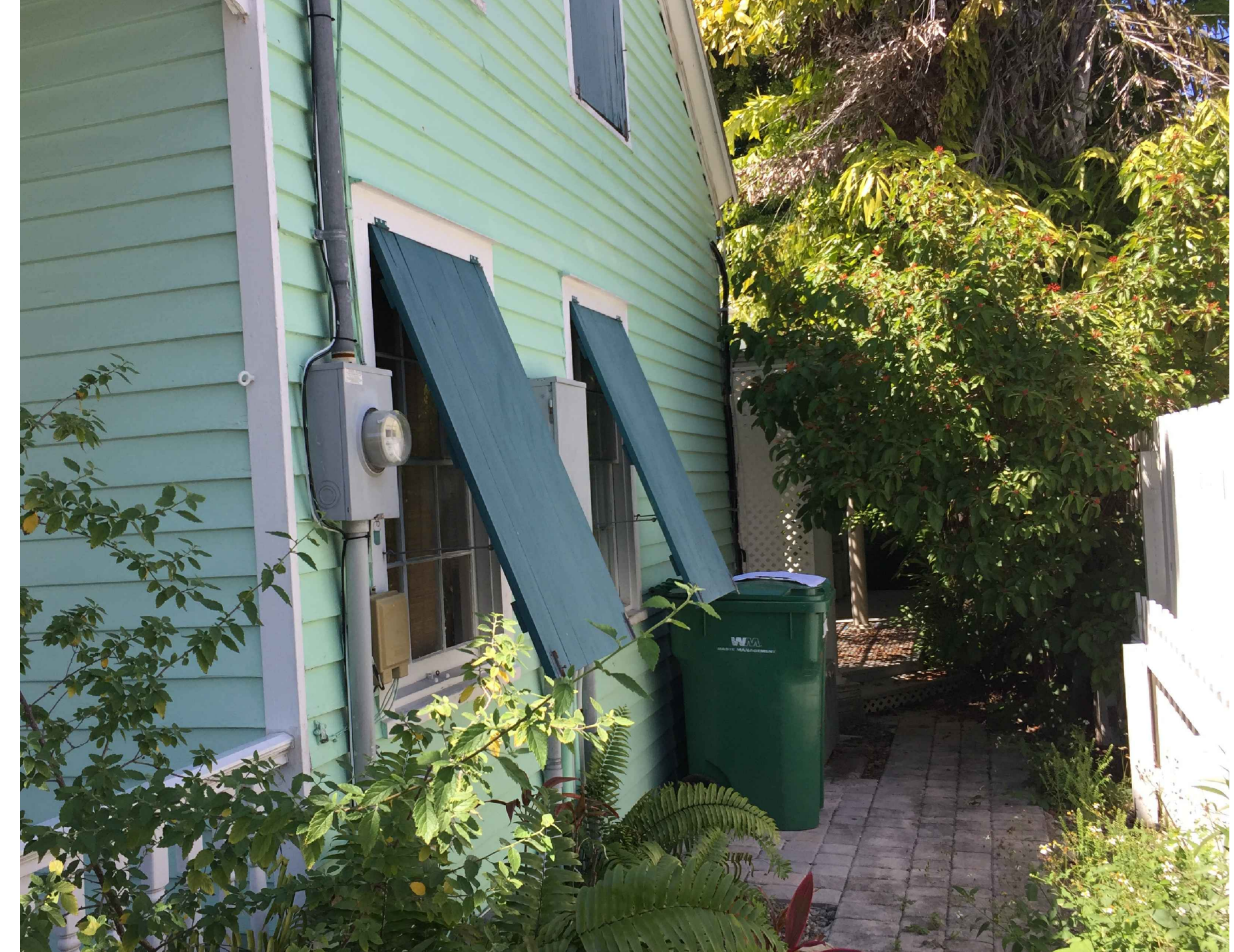
4 PHOTOGRAPH OF EXISTING EAST ELEVATION
