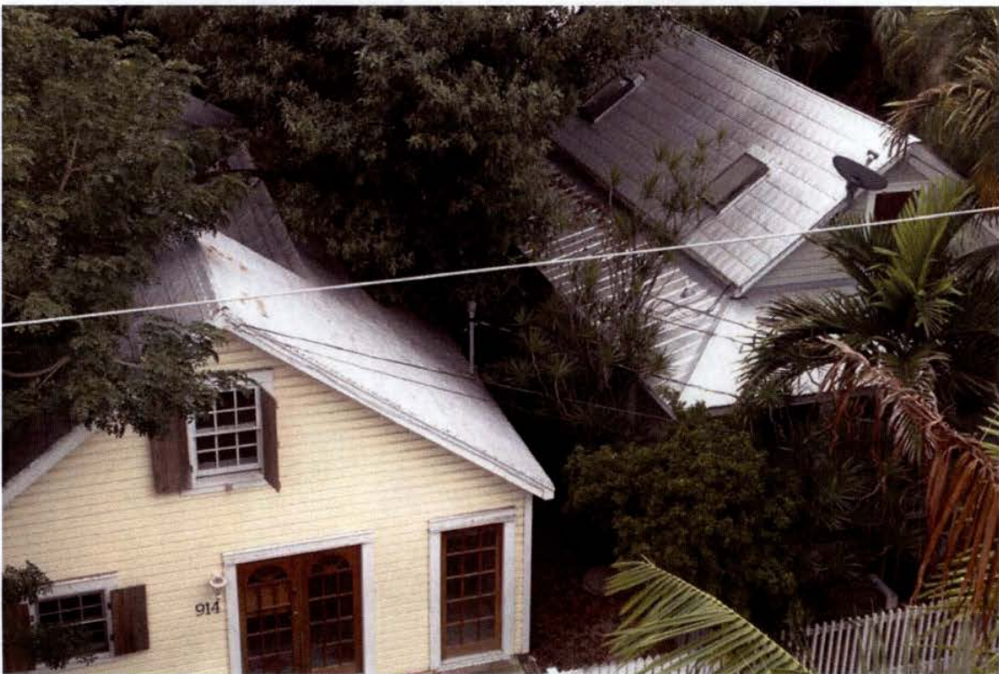
FRONT ELEVATION & NEIGHBORING STRUCTURE
