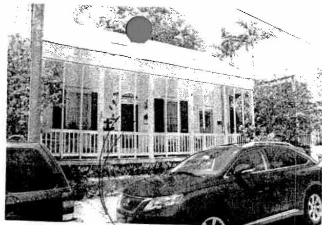
REMOVE ALL SCREEN FRAMING ON HISTORIC PORCH (W&S IN ES)
