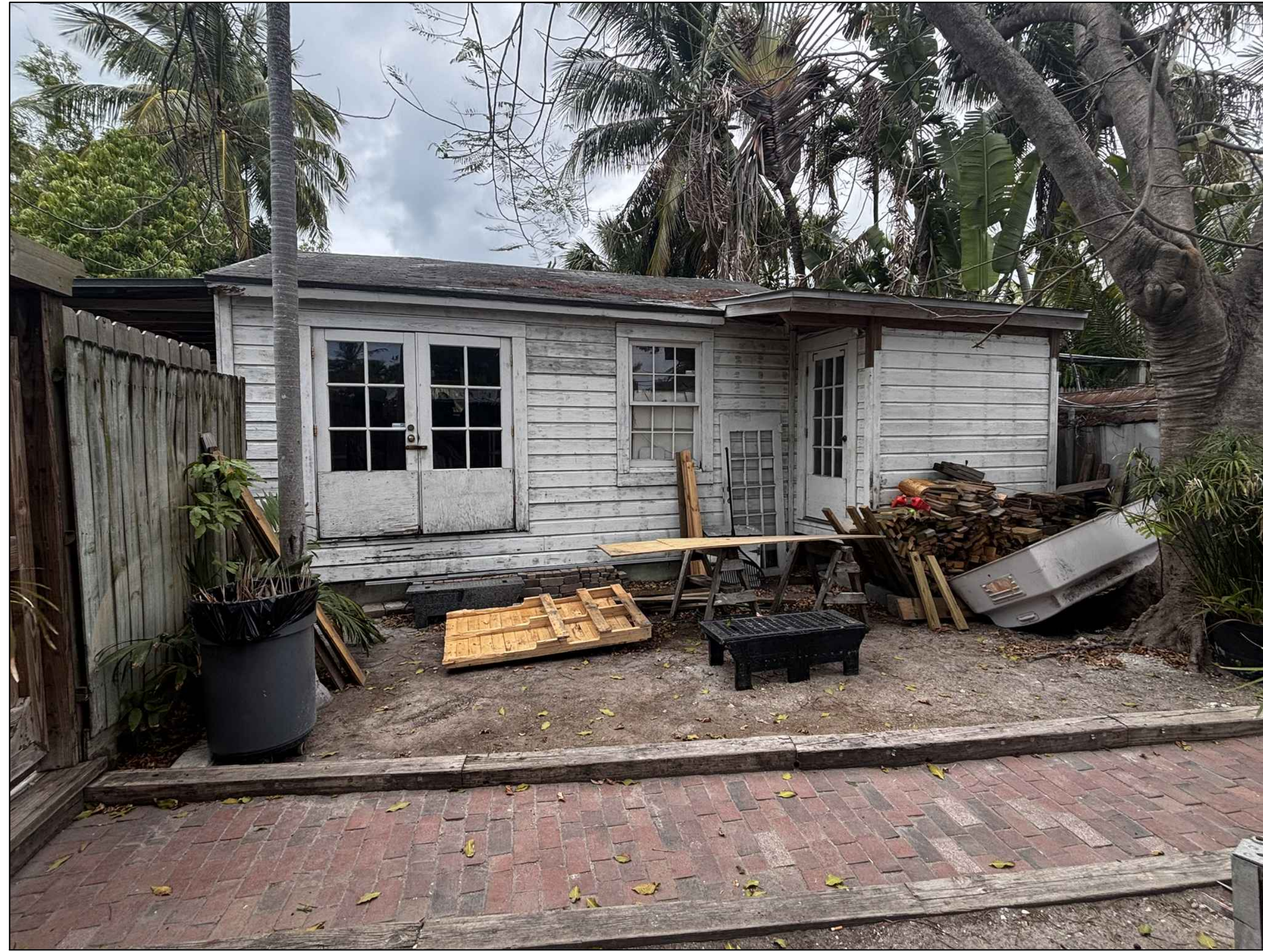
1 VIEW FROM SOUTH SIDE OF THE PROPERTY A6 SCALE: N.T.S.
