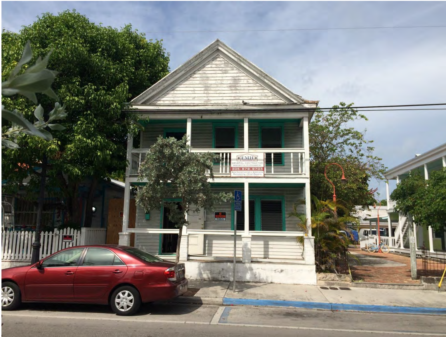
FRONT VIEW FROM WHITEHEAD ST.
