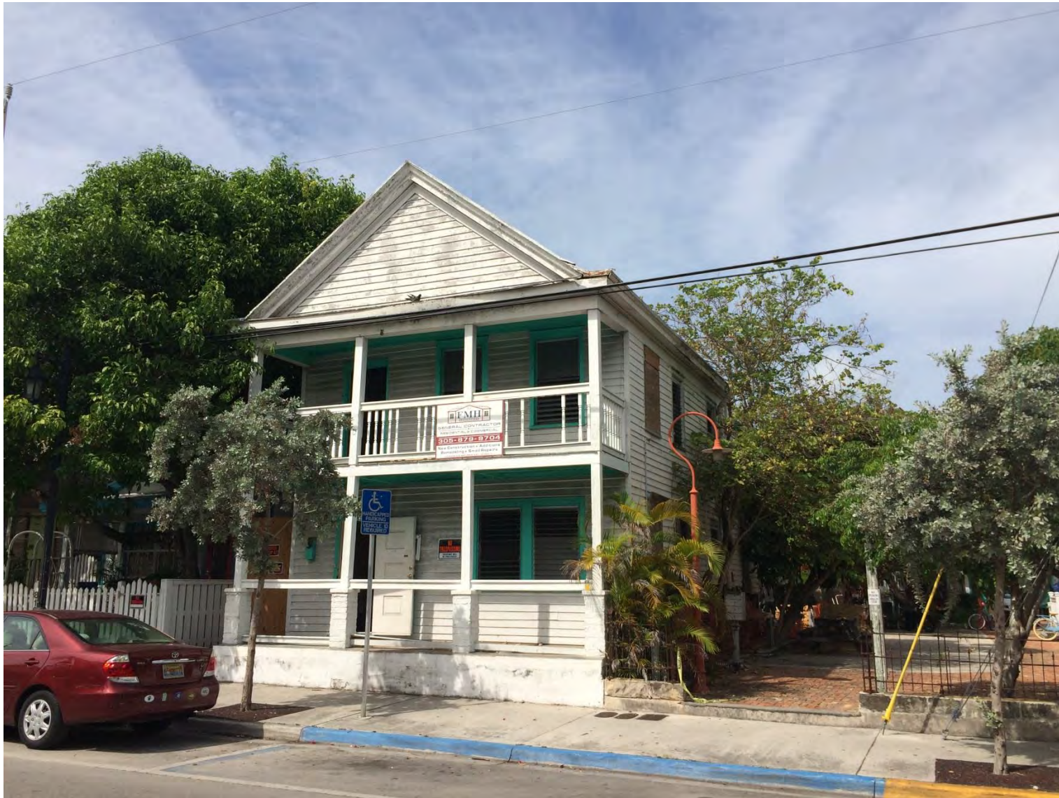
RIGHT SIDE VIEW FROM WHITEHEAD ST.
