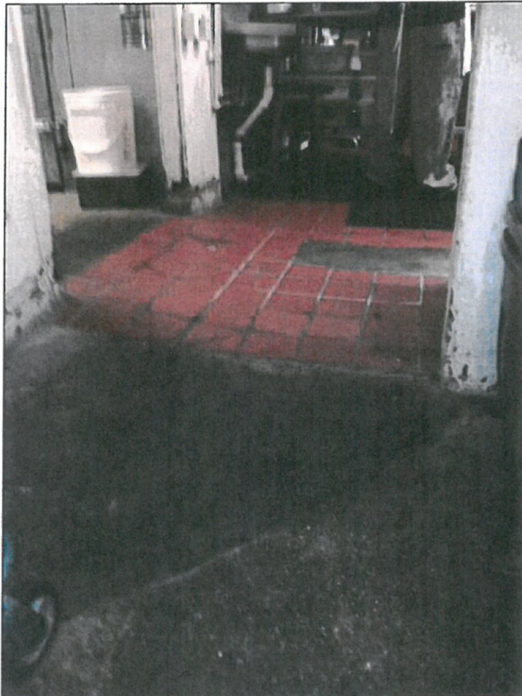
6.2 Picture 5 Typical Flooring Situation
