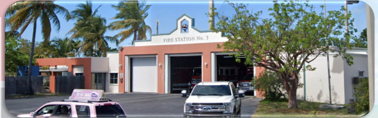
EXISTING FIRE STATION 3
