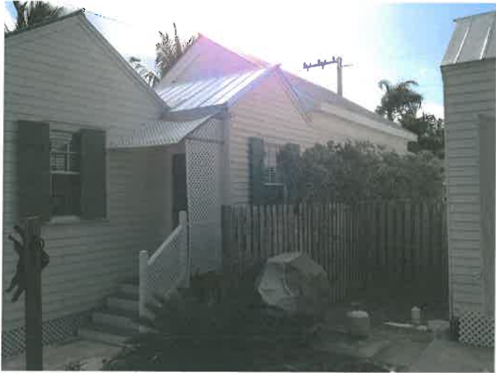
REAR VIEW (AREA TO BE ENCLOSED)
