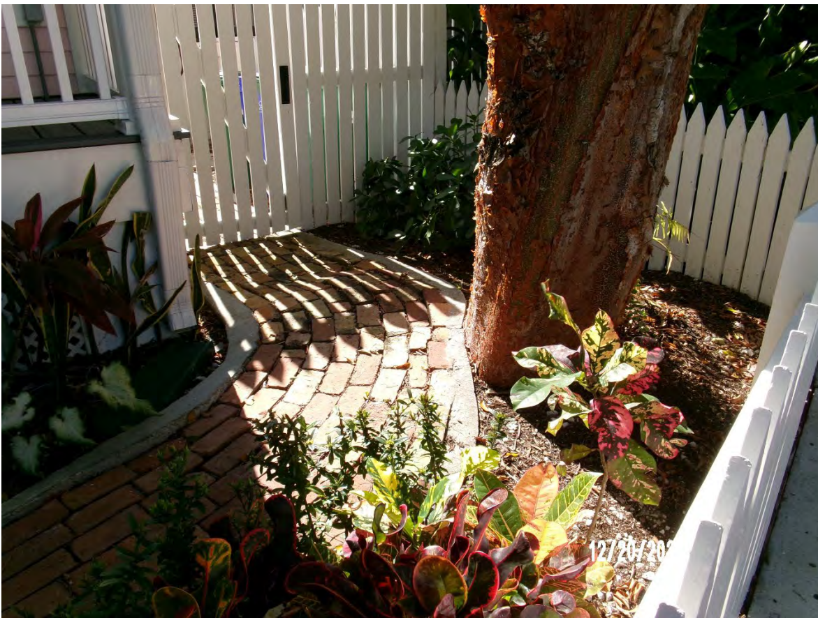
Photo of base of tree area. Pavers installed a few years ago placed too close to base of tree.
