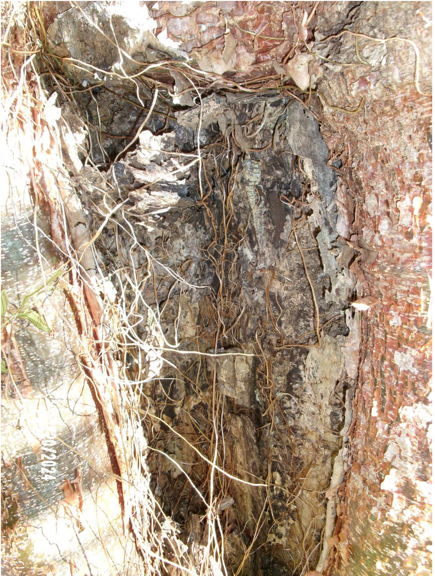
Close up photo of trunk decay/old damage area. No evidence of live insects during inspection.
