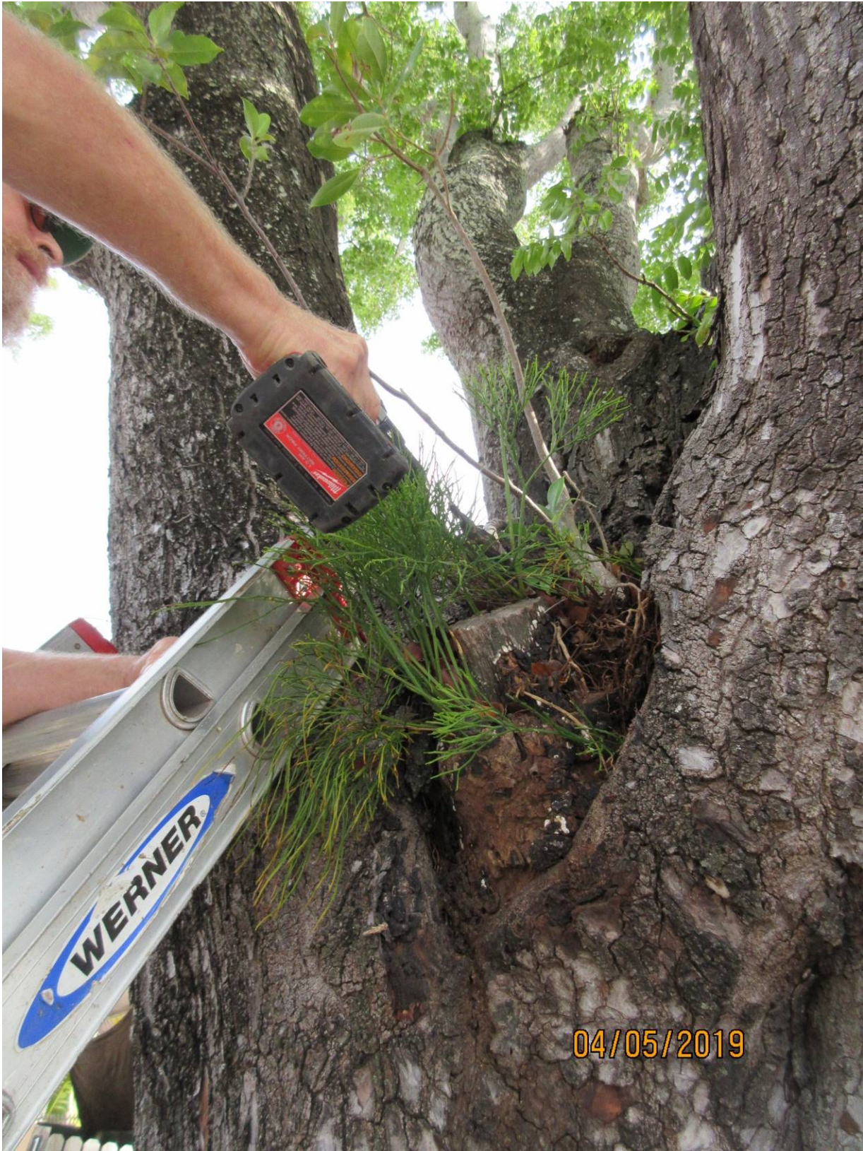
Drill location above: drill bit easily into the wood-10" soft wood
