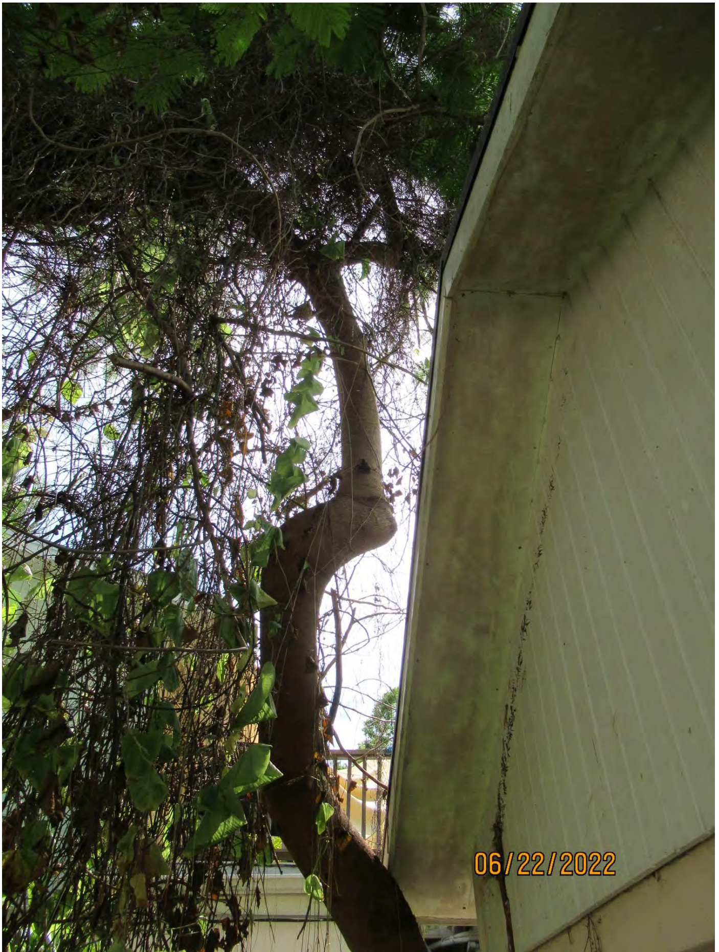
Photo showing tree trunk and canopy, view 4.
