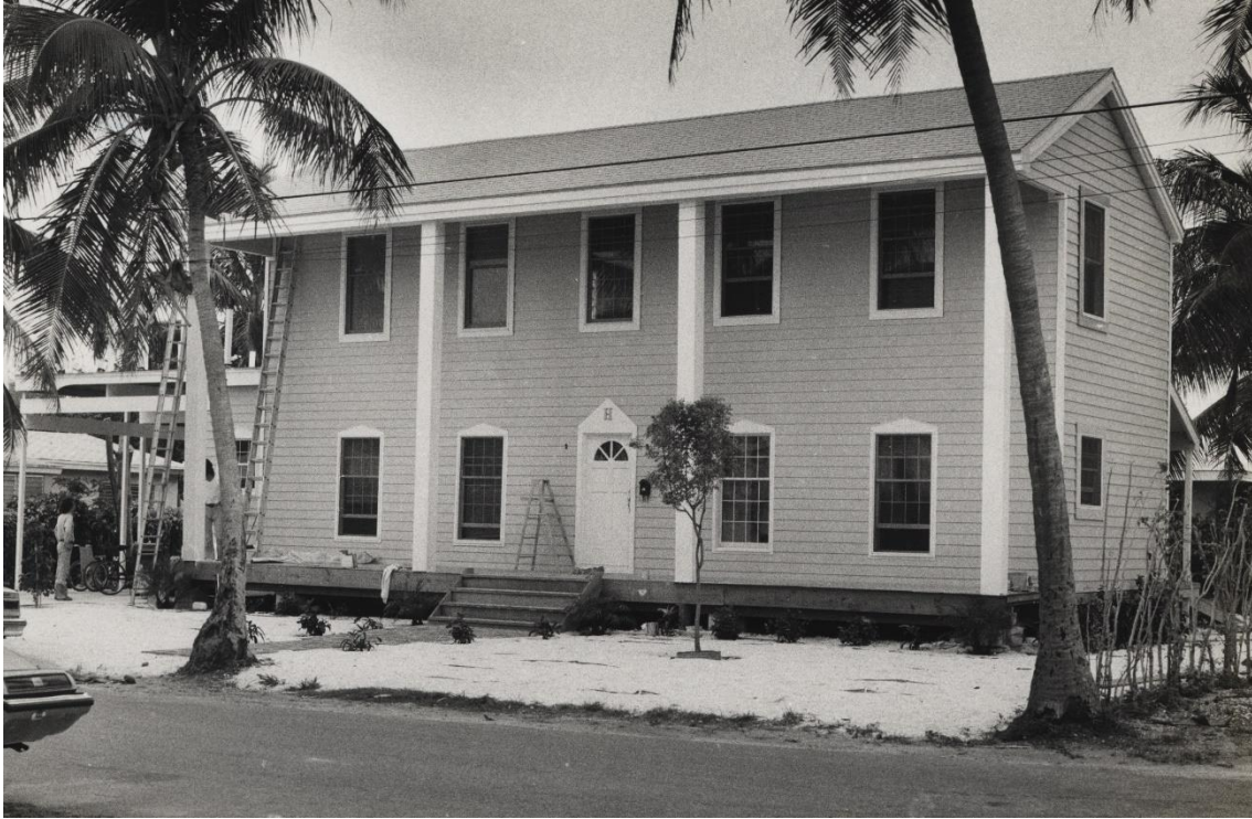
House in 1970 while roof deck was under construction. Monroe County Library.
