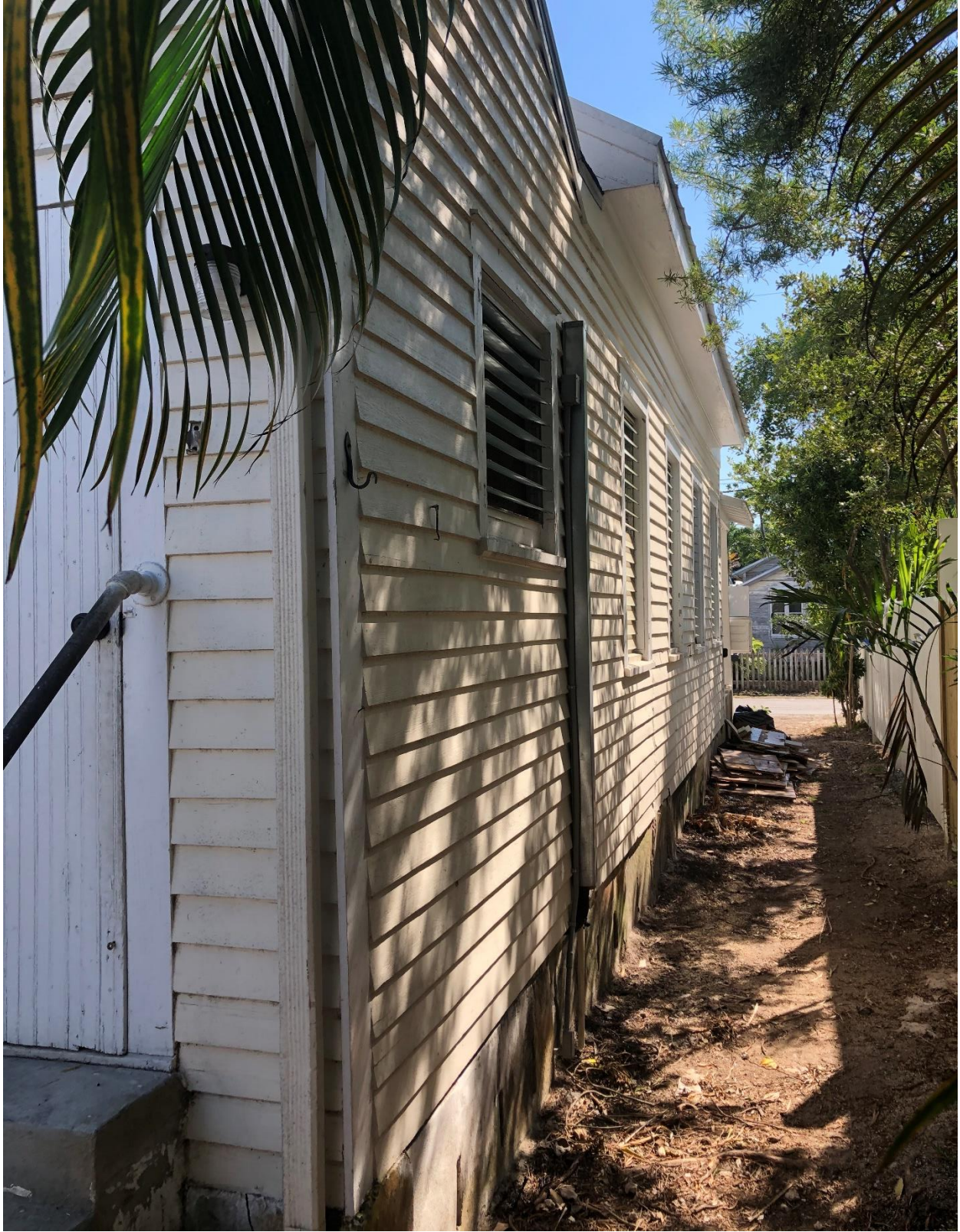
Photo of 1311 Eliza Street. Back West Side View.
