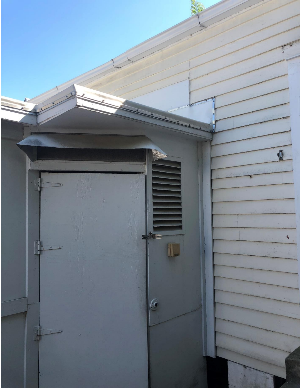
Photo of 1311 Eliza Street. Back Addition.
