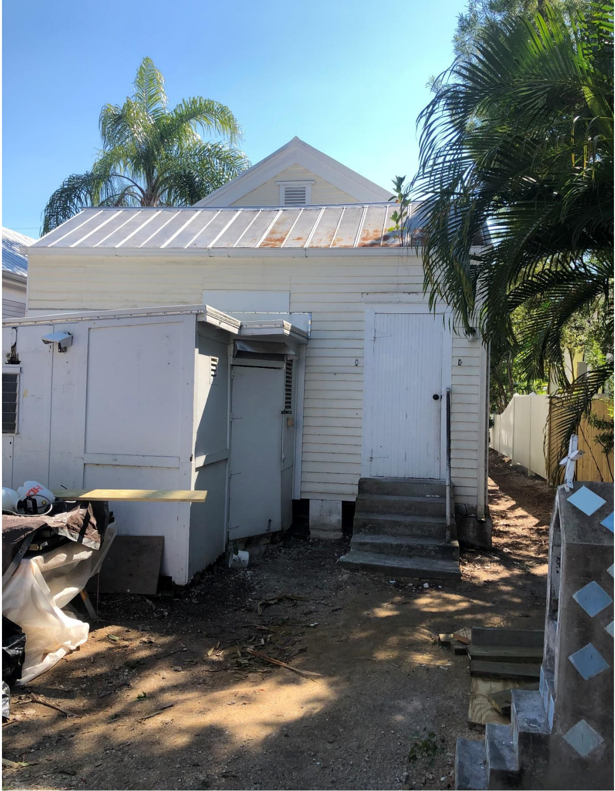
Photo of 1311 Eliza Street. Rear View.
