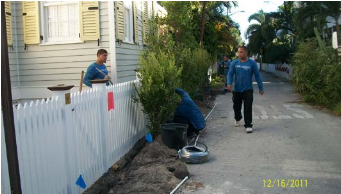
405 Frances Case # 11-1506 Fence encroaching on city's row
