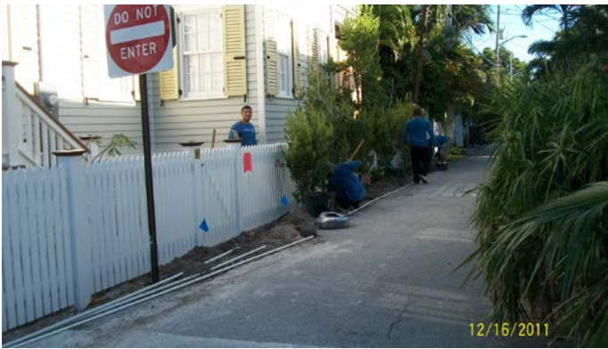
405 Frances Case # 11-1506 Fence encroaching on city's row
