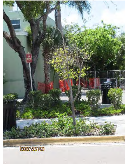
Tree #20 to be removed and replaced.
