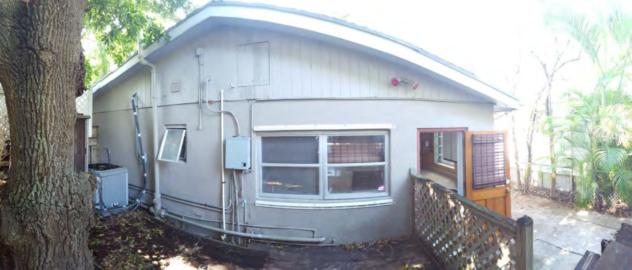
Rear of Front Building
