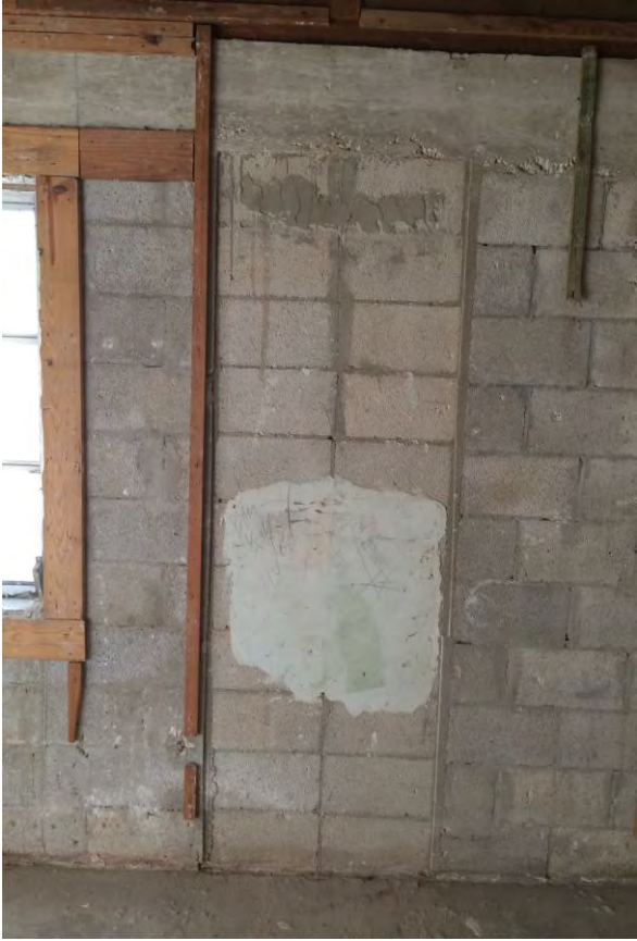
Pre-existing door opening
