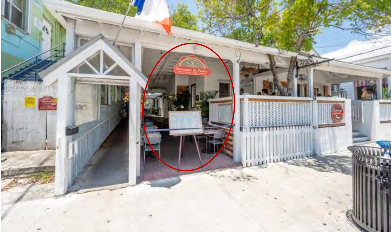
Photo of Area Under Review Before Current Renovations.
