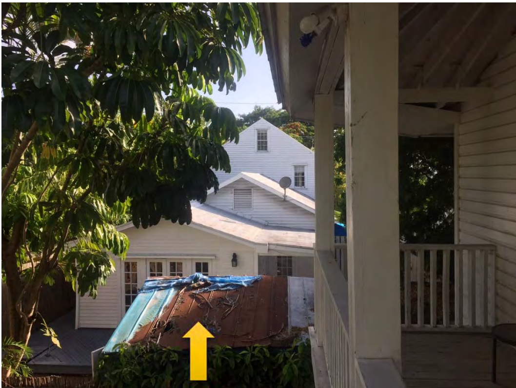
NEIGHBOR TO REAR AT WEST
