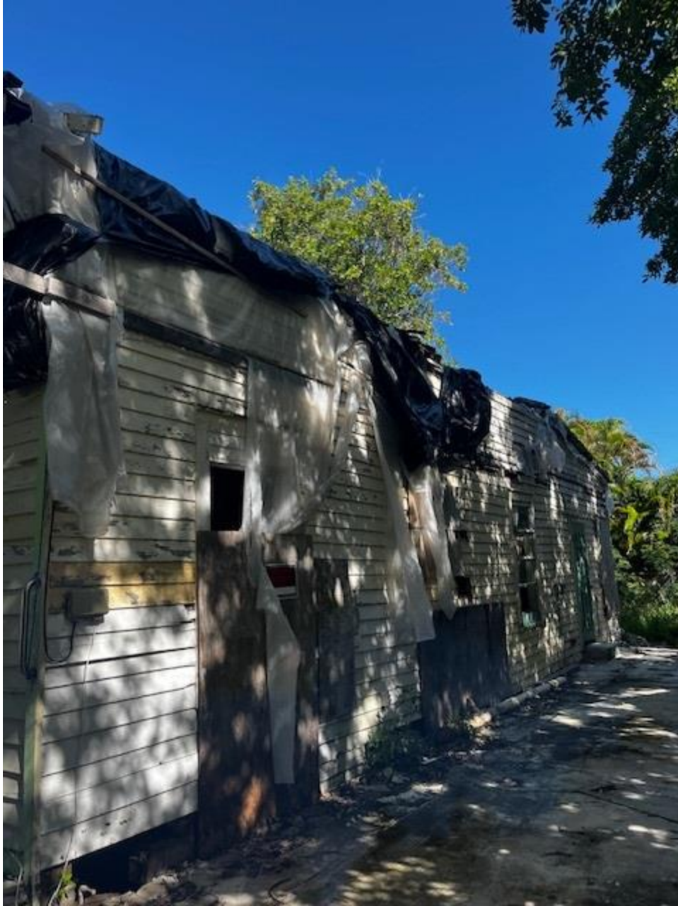
Current conditions at south elevation.
