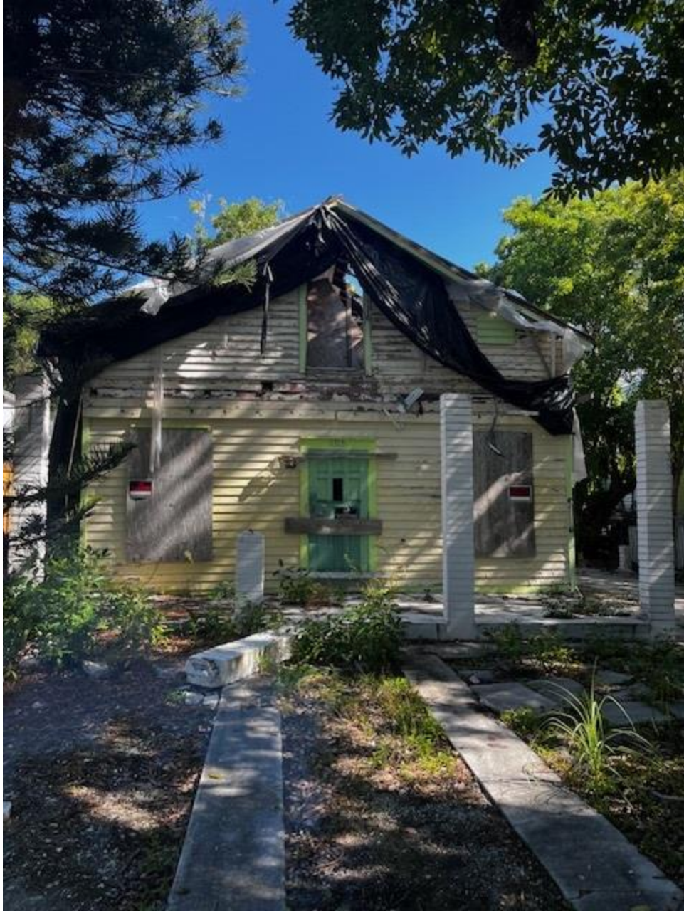
Current conditions at front (west) elevation.
