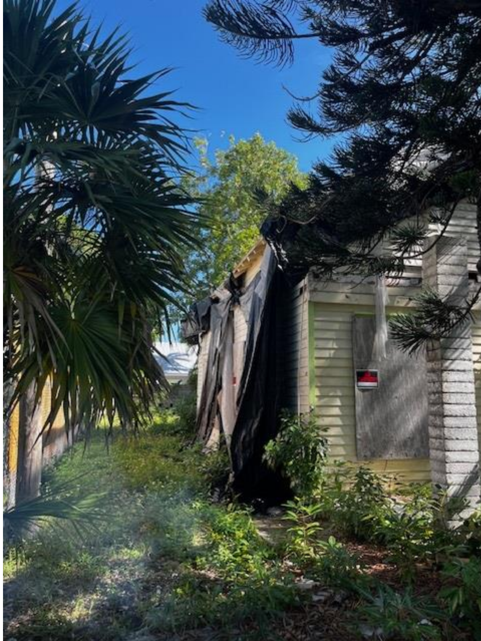
Current conditions at north elevation.
