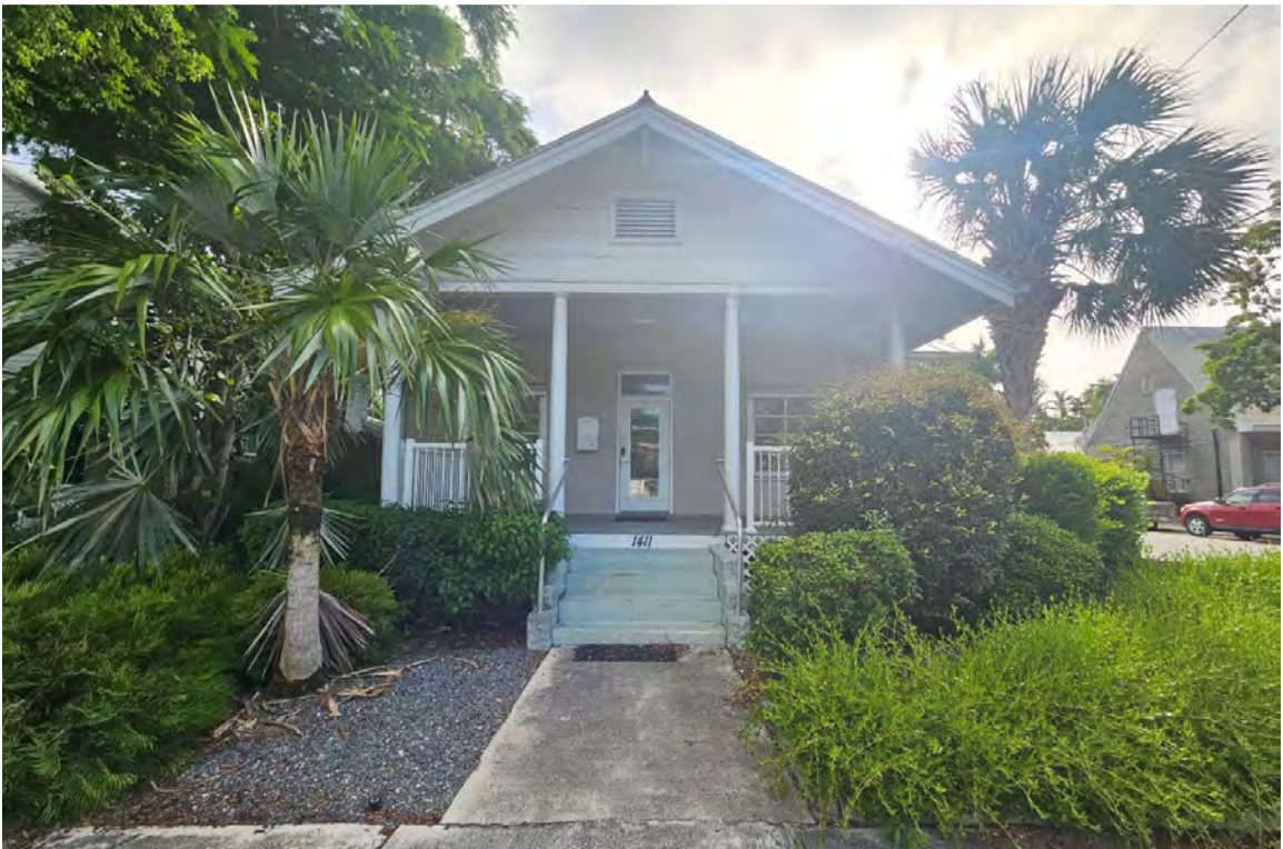
Current photo of house under review.
