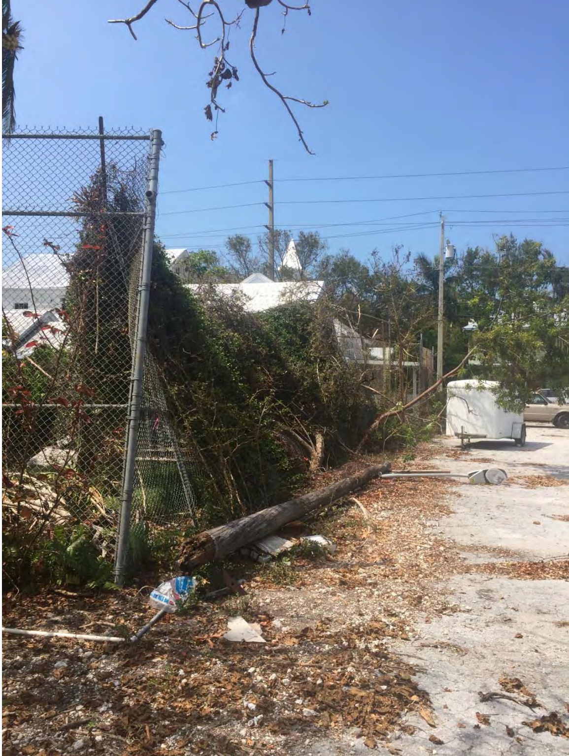
DAMAGED FENCE – HURRICANE IRMA SEPT. 2017
