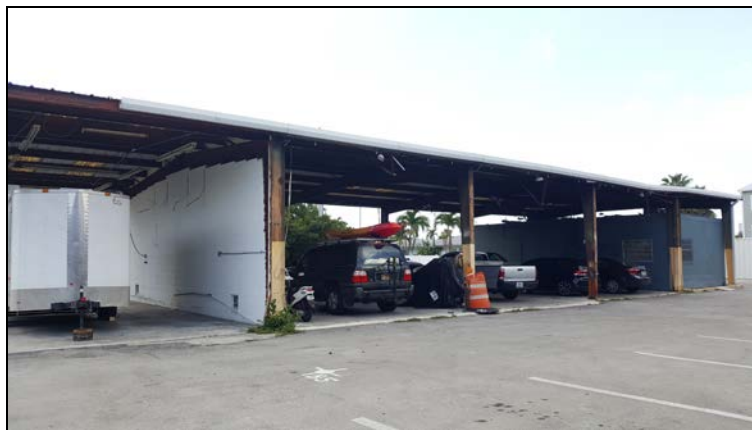
Image of the parking canopy with small structure at one end to be removed.
