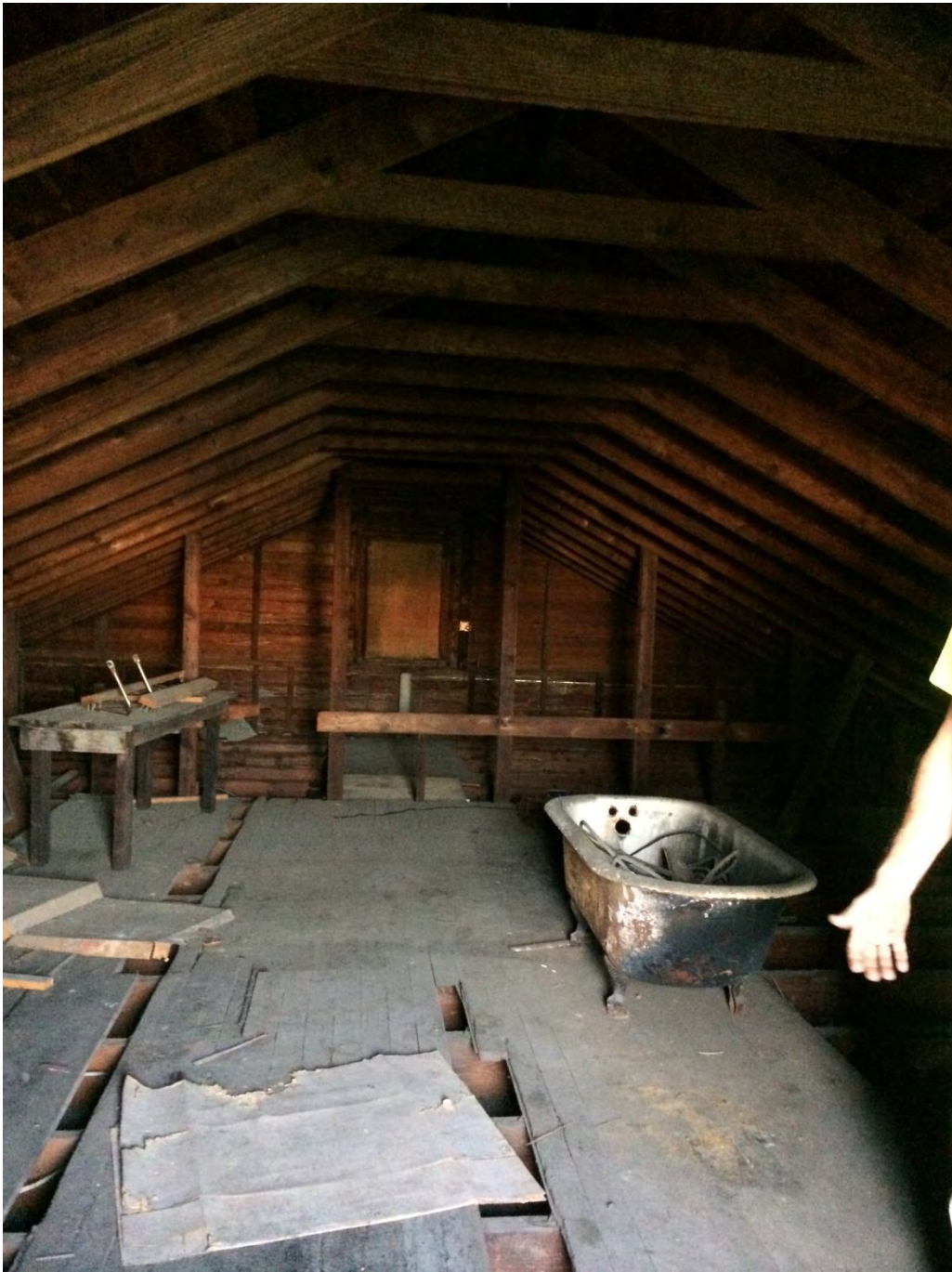
Photo: Existing Conditions; Attic Facing Bagatelle
