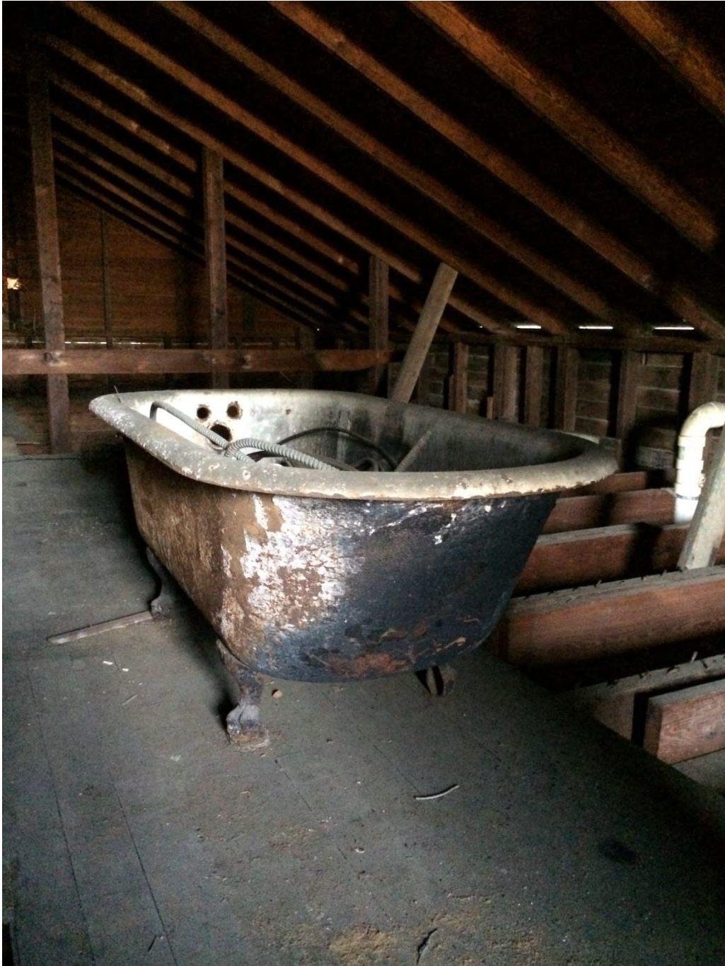
Photo: Existing Conditions; Original Clawfoot Bathtub
