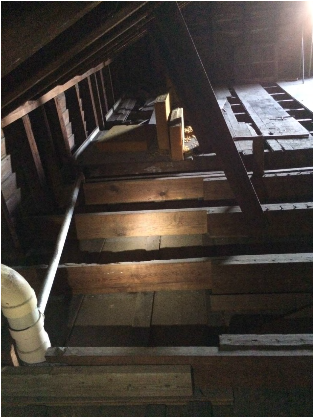
Photo: Existing Conditions; Original Stair Opening
