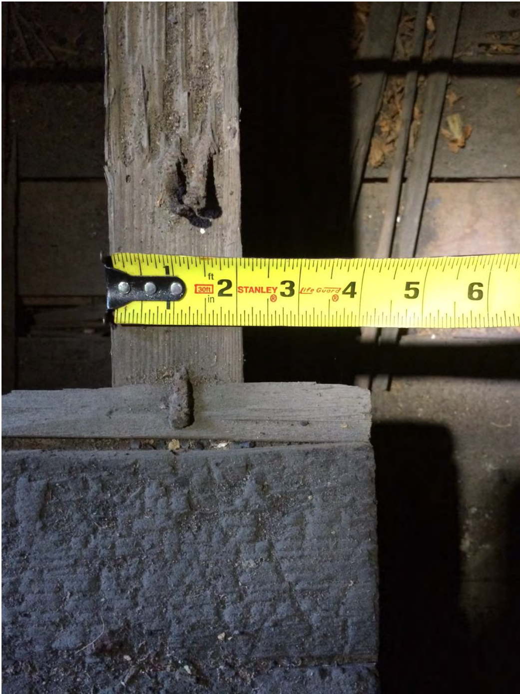
Photo: Existing Conditions; Original 2" Lumber
