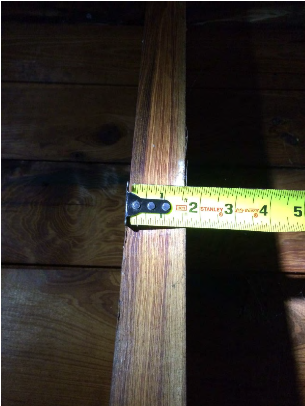
Photo: Existing Conditions; New 1-1/2" Nominal Lumber
