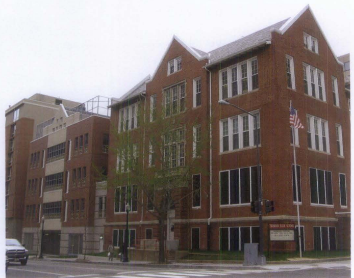
Figure 3. The red and buff-colored parking addition with a rooftop playground is compatible with the early-20th century school as well as with the neighborhood in which it also serves as infill in the urban setting.
