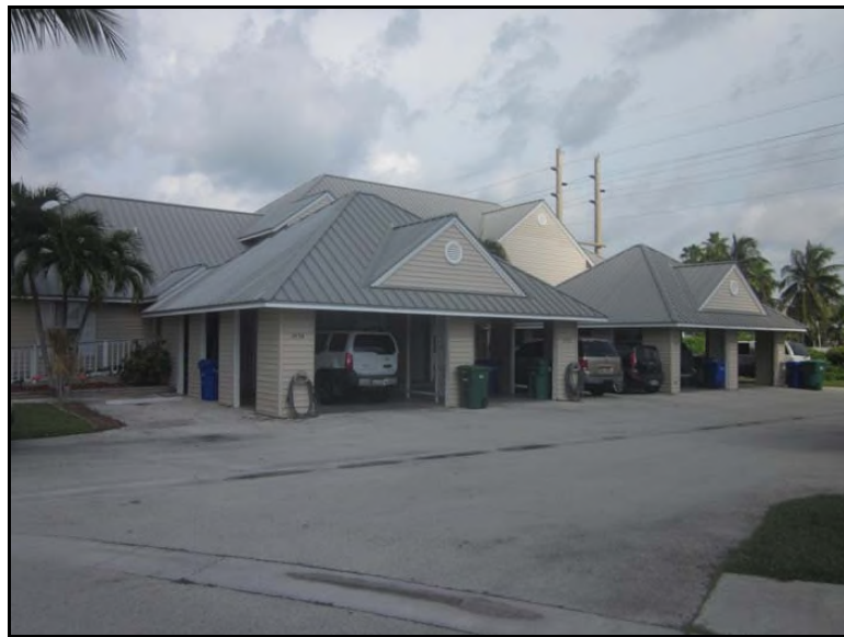
View of Housing Complex Units
