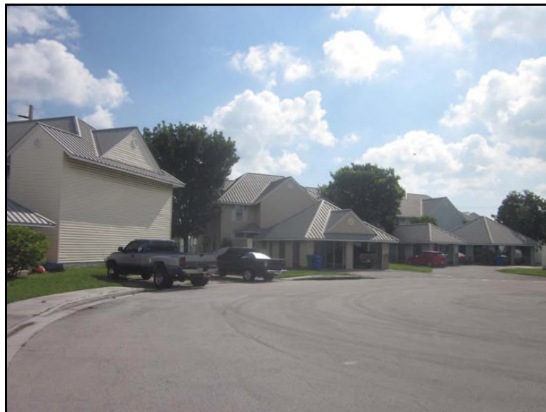
View of Housing Complex Units
