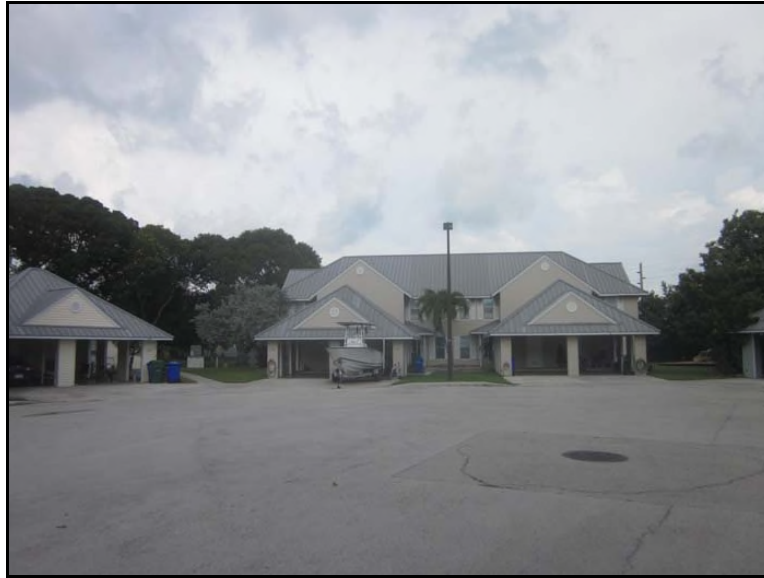
View of Housing Complex Units
