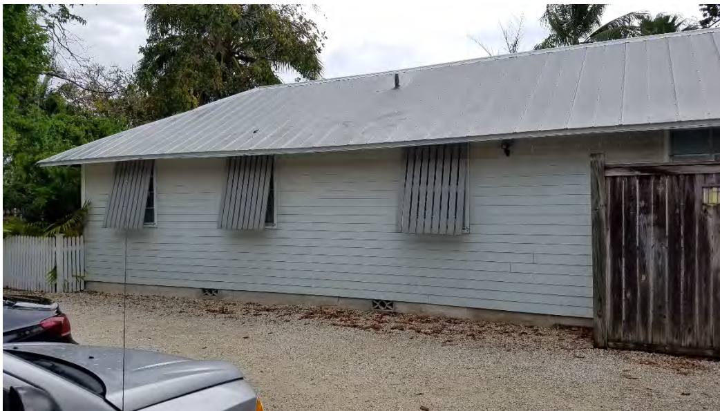
VIEW NORTH EAST - Back side of Key Lime Inn original Motor Lodge.
