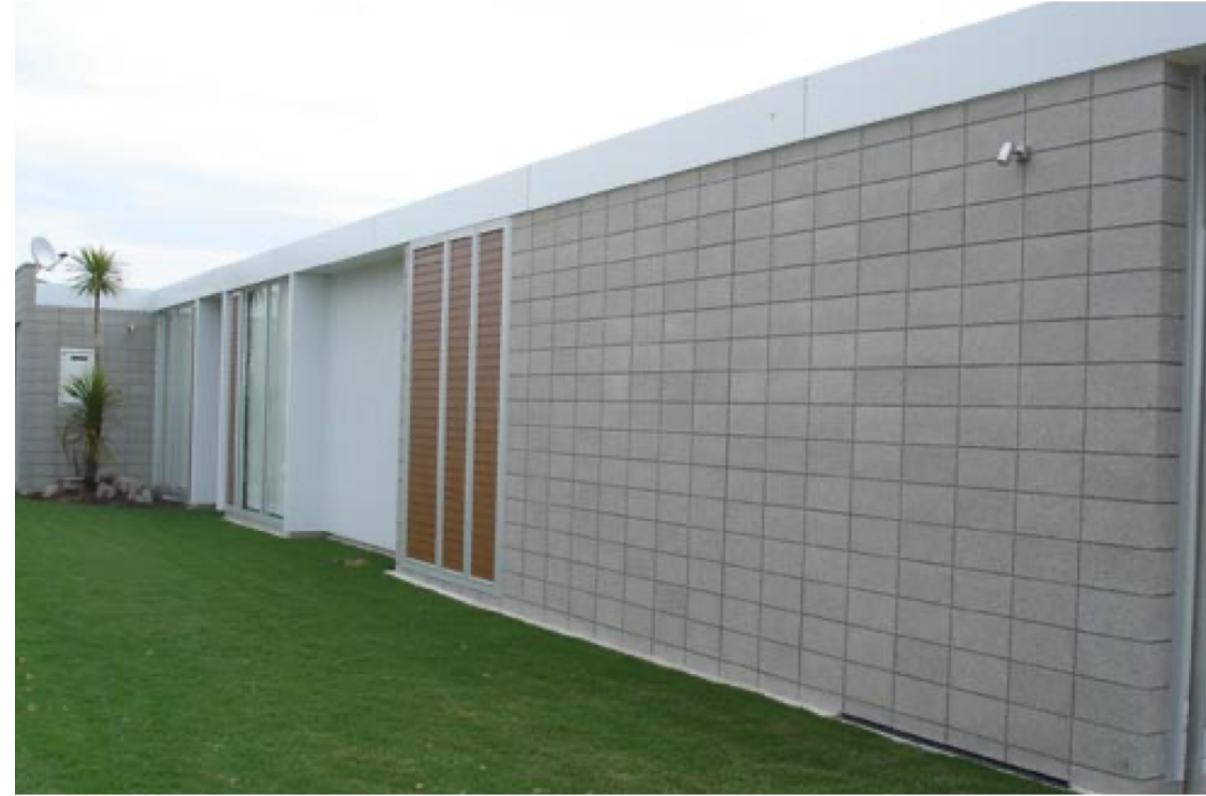
STUCCO FINISH OVER CMU - STACK BOND PATTERN
