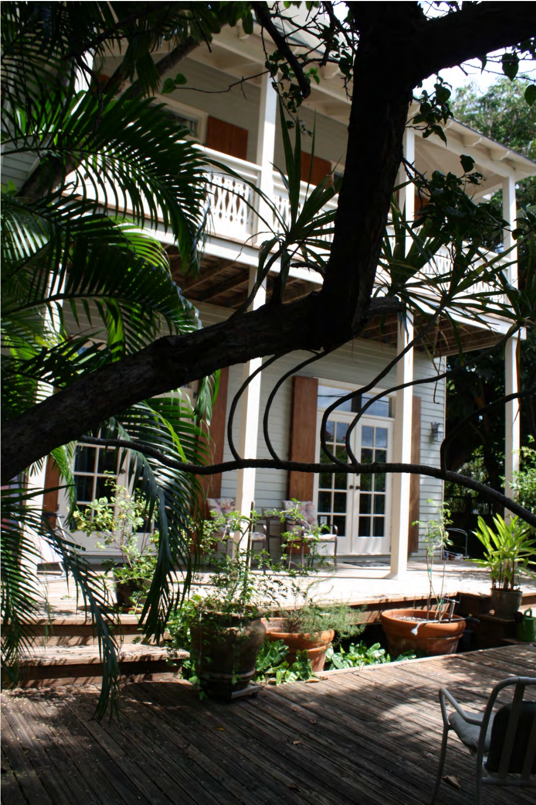
Façade facing United Street
