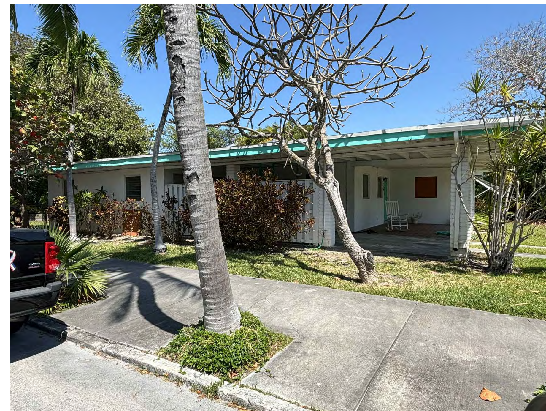
1 A8 VIEW FROM SIDE OF THE HOUSE (EXISTING WEST ELEVATION) SCALE: N.T.S.
