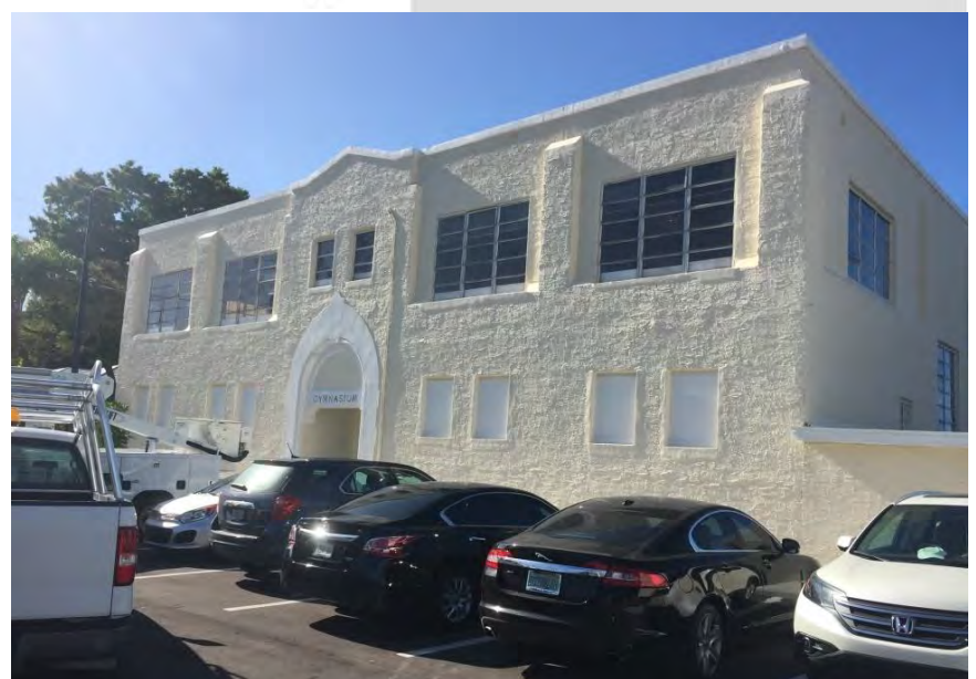
EXISTING BUILDING PRIOR TO CONSTRUCTION
