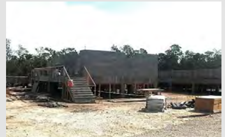
CATHOLIC CHARITIES UNDER CONSTRUCTION
