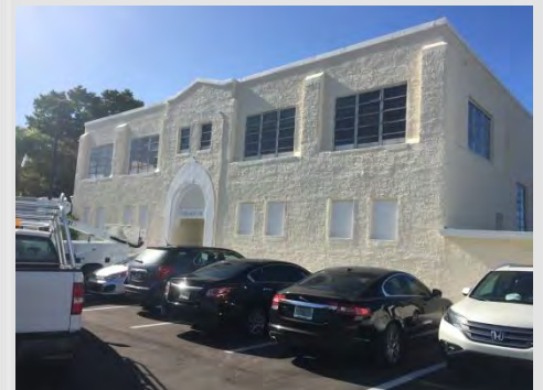
OLD GYMNASIUM BUILDING
