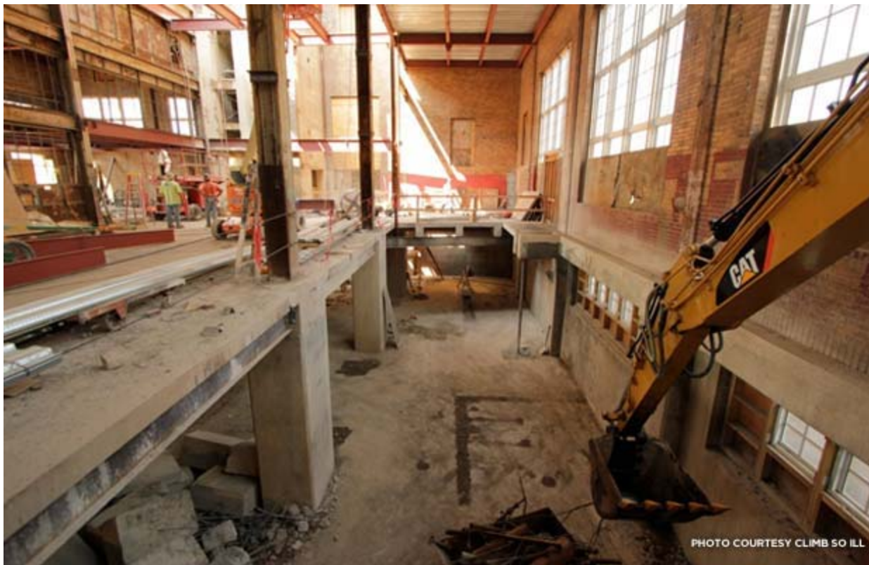
Construction during renovation.
