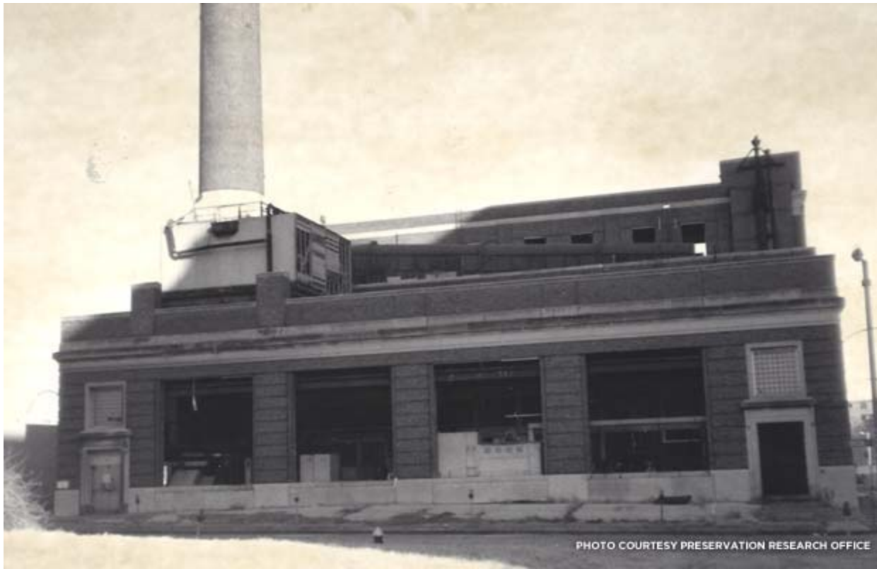
The Power Plant's windows were missing by 1994.
