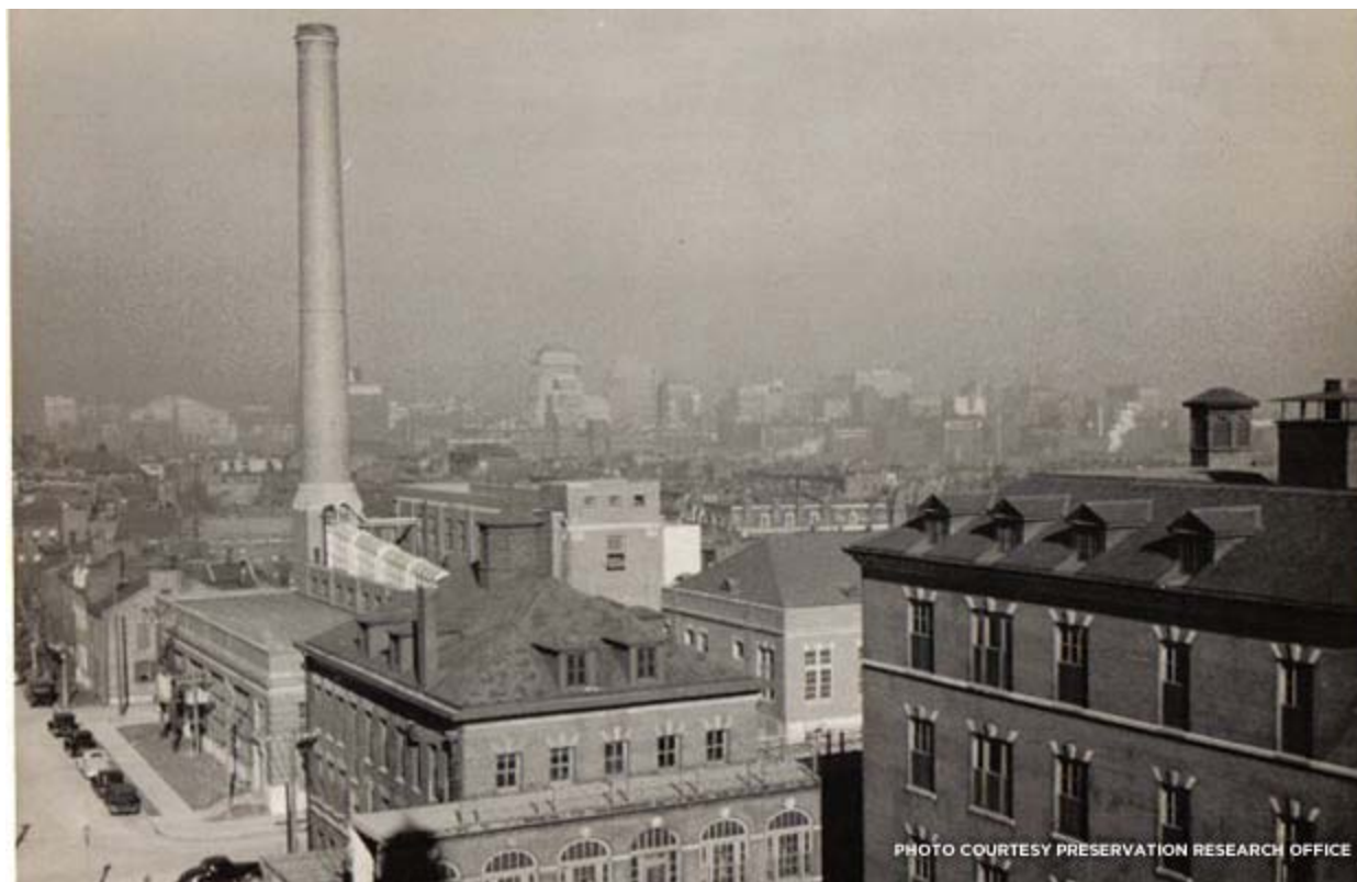
View toward the Power Plant during the City Hospital modernization project.
