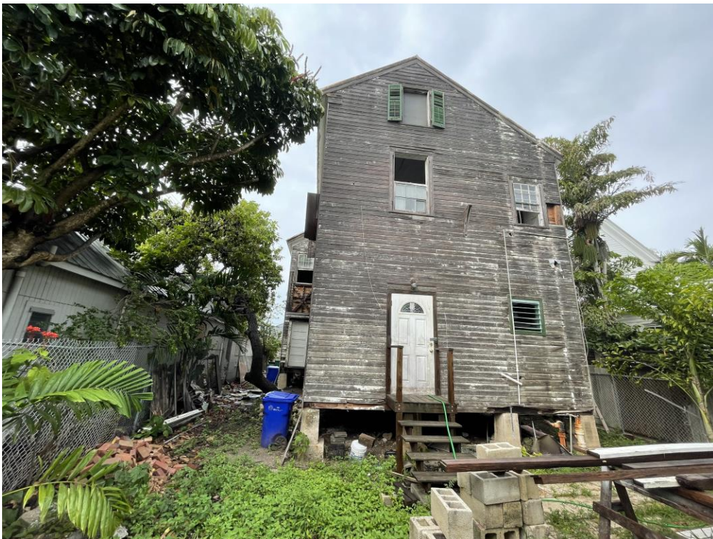
Rear View with Southern & Northern Properties
