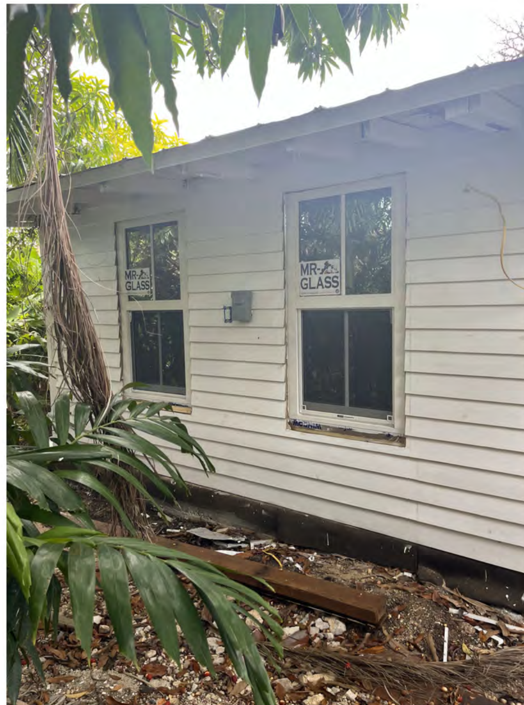
CURRENT REAR OF HOUSE, NEW ADDITION
