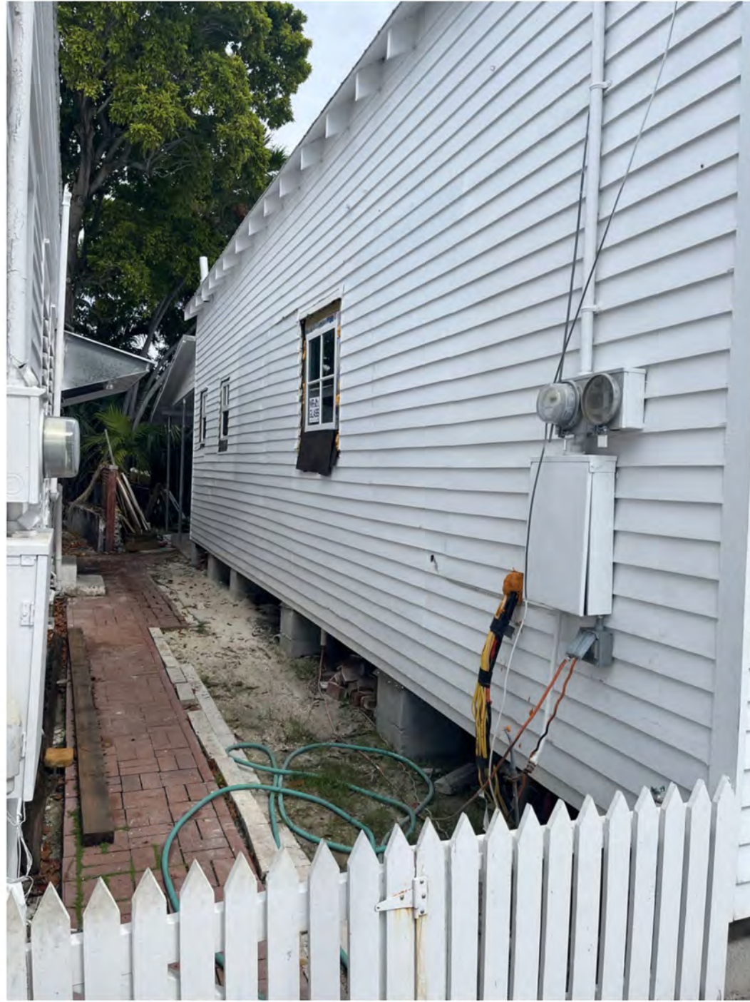
CURRENT NORTH SIDE FACADE, FACING REAR
