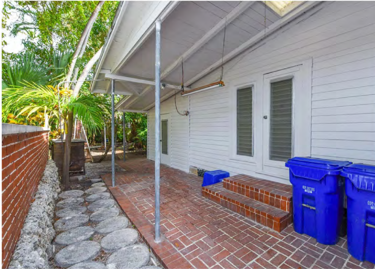
PREVIOUS REAR FACADE, AT NON-HISTORIC ADDITION
