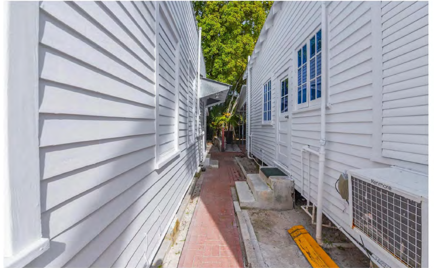
PREVIOUS NORTH SIDE FACADE, FACING REAR
