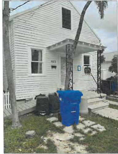
1 FRONT FACADE A0.2 REFURBISHED 2 OVER 2 WINDOWS FROM REAR OF HOUSE.
