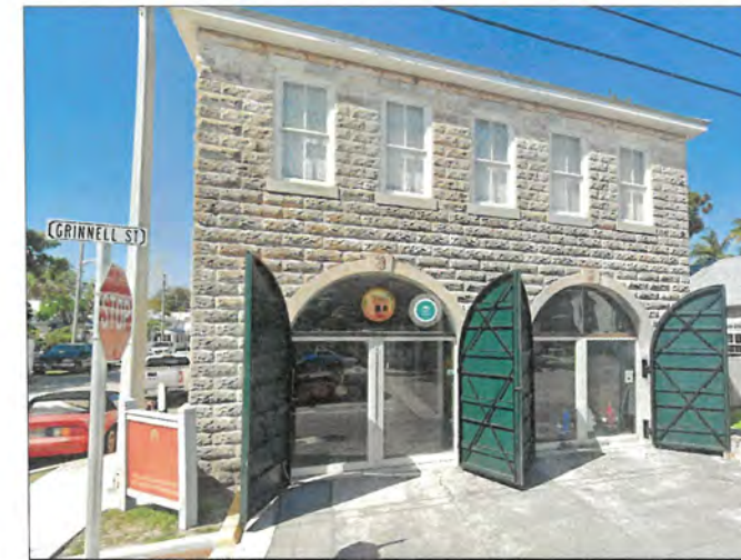
11 NEIGHBORING PROPERTIES A0.2 HISTORICAL FIRE HOUSE MUSEUM EXAMPLE OF EXISTING 2 OVER 2 WINDOWS
