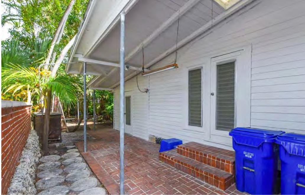
Exterior wall prior to alteration.
