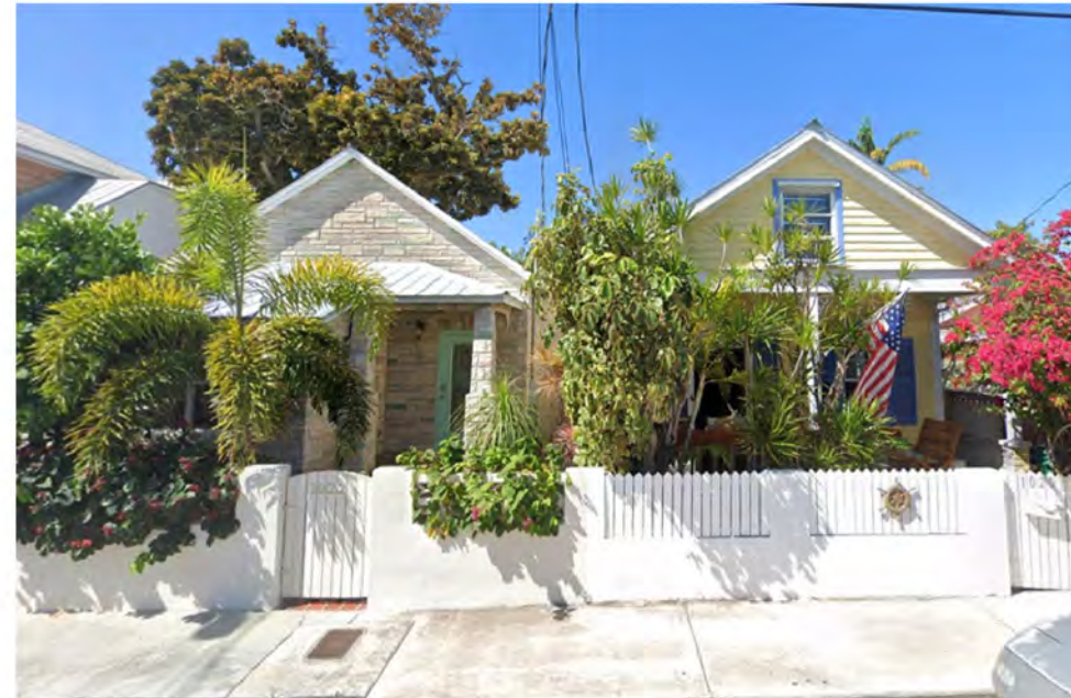
1020, 1022 GRINNELL EXAMPLE OF 2 OVER 2 WINDOWS ON PRIMARY FACADE
