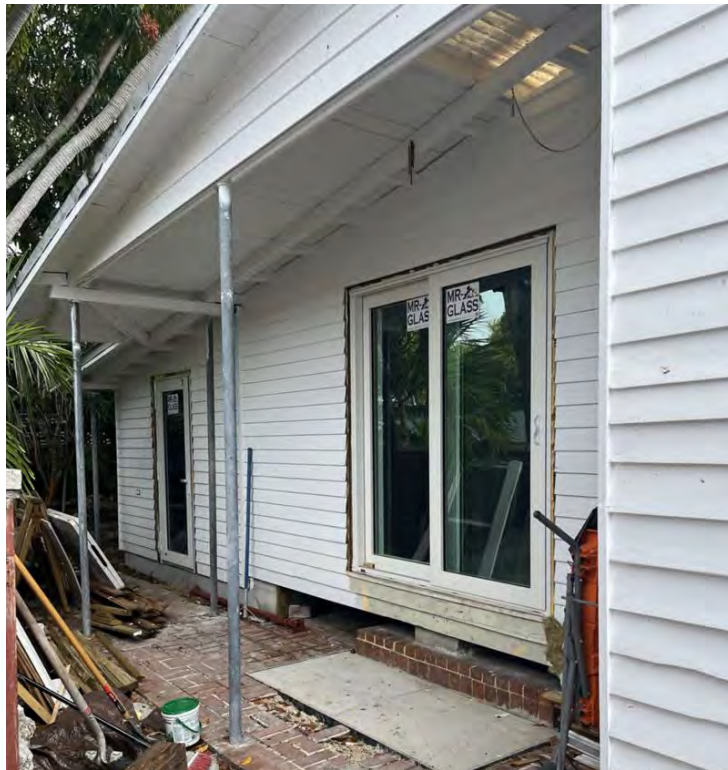
Exterior wall after alteration.
