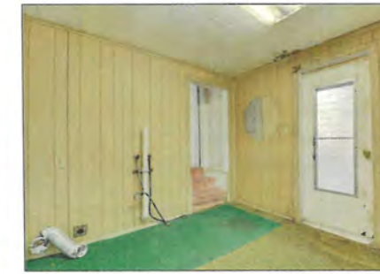
20 BACK ROOM A0.1 PREVIOUS INTERIOR
