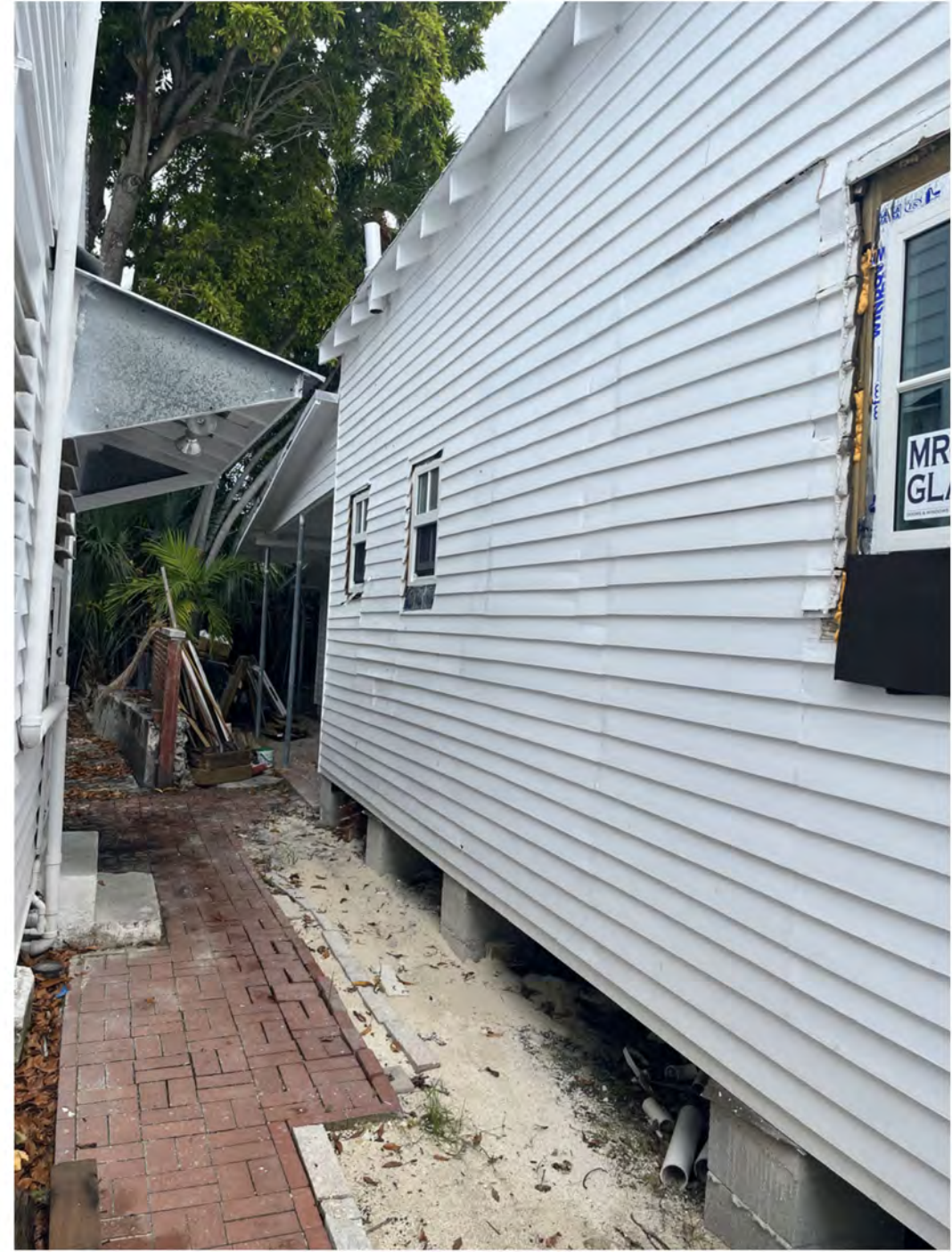
CURRENT NORTH SIDE FACADE, FACING REAR
