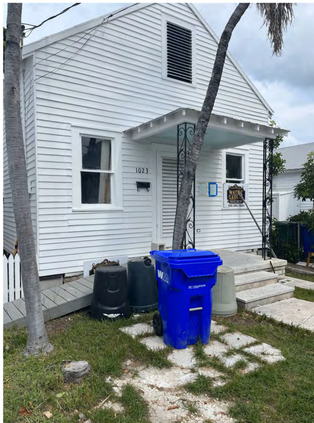
CURRENT FRONT FACADE
