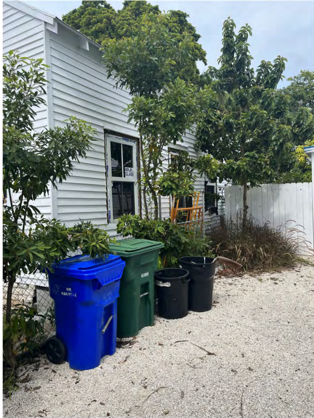
CURRENT SOUTH SIDE FACADE, FACING REAR
