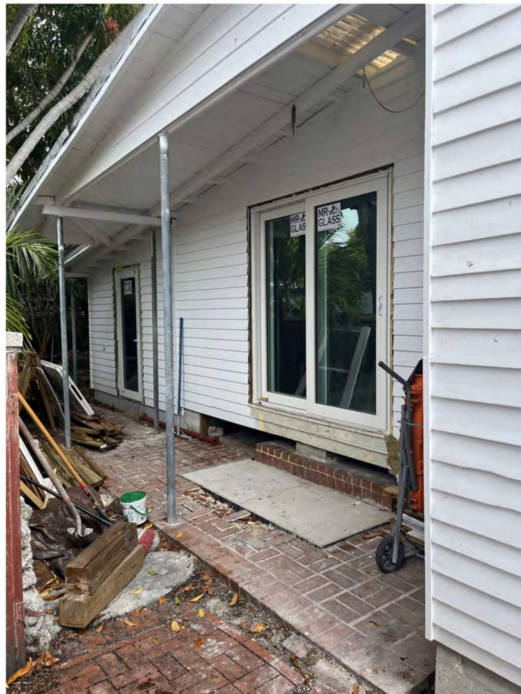
CURRENT REAR OF HOUSE, NEW ADDITION
