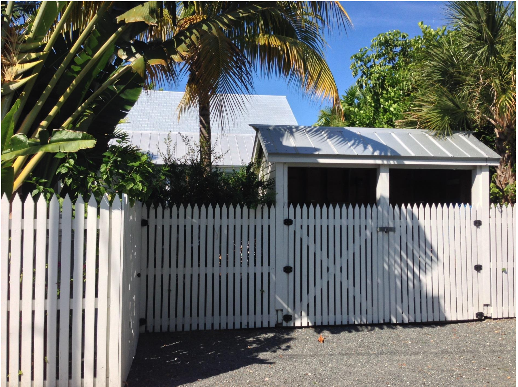
Rear of house. Existing shed structure that holds mechanical equipment.
