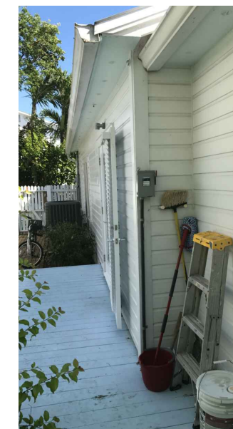
EXISTING N. SIDE OF HOUSE FROM REAR
