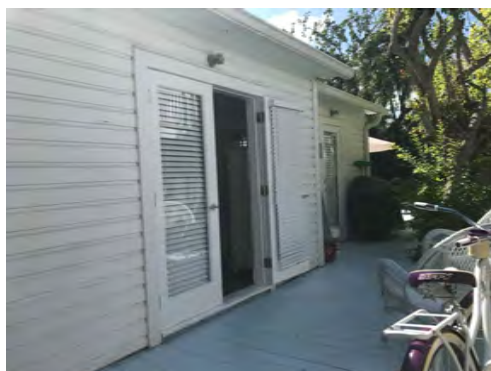
EXISTING N. SIDE OF HOUSE FROM FRONT
