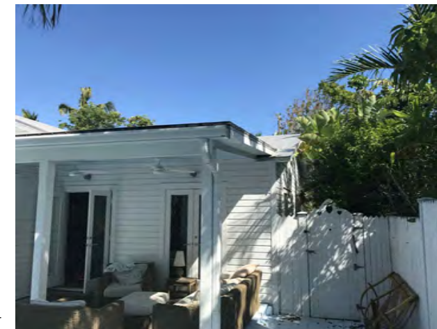
EXISTING S. SIDE OF HOUSE FROM REAR
