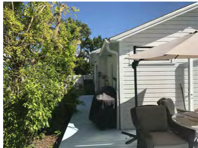
EXISTING N. SIDE OF HOUSE FROM REAR
