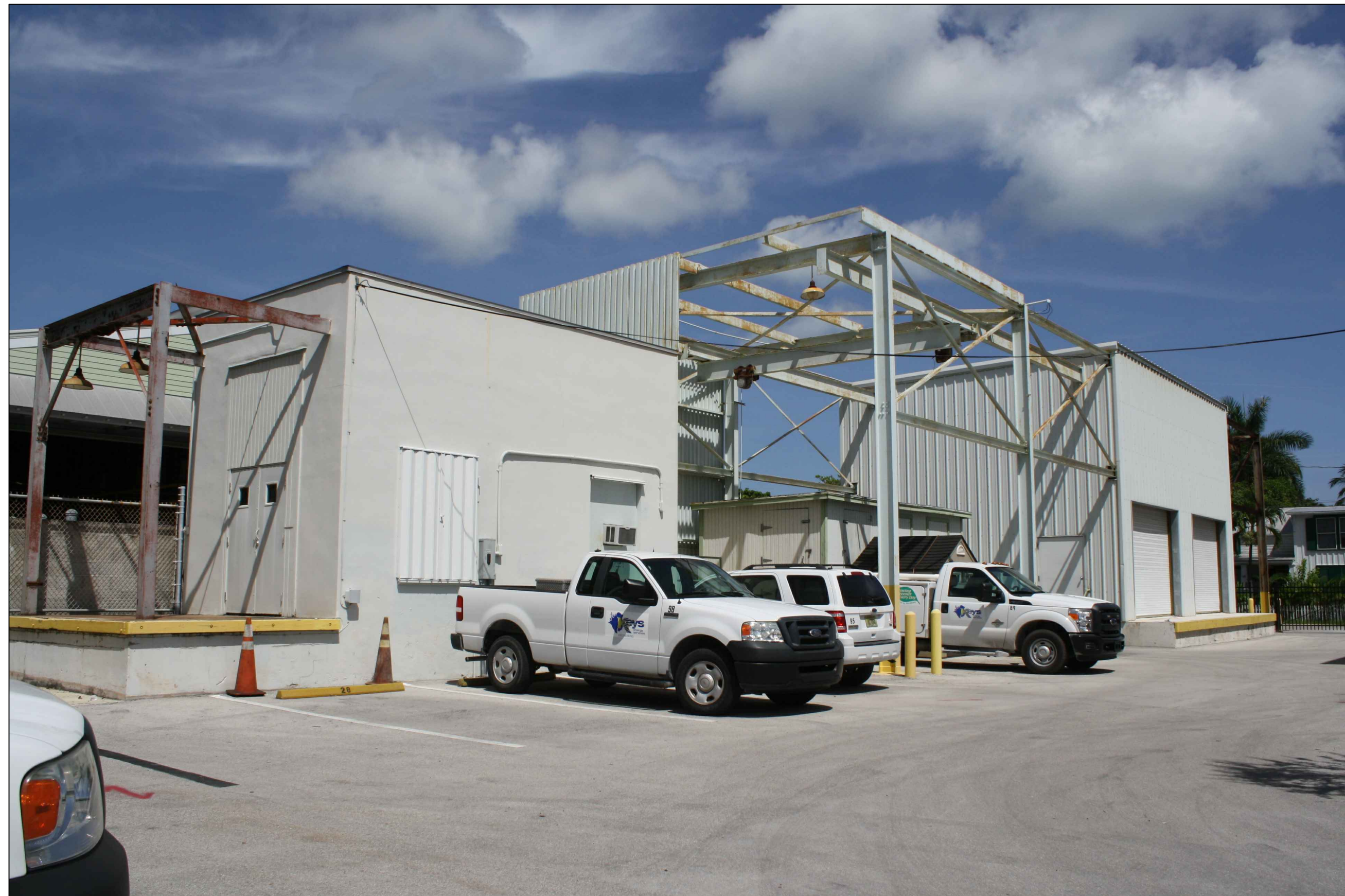
2 H3 STORAGE SHEDS ON EAST SIDE OF SITE
