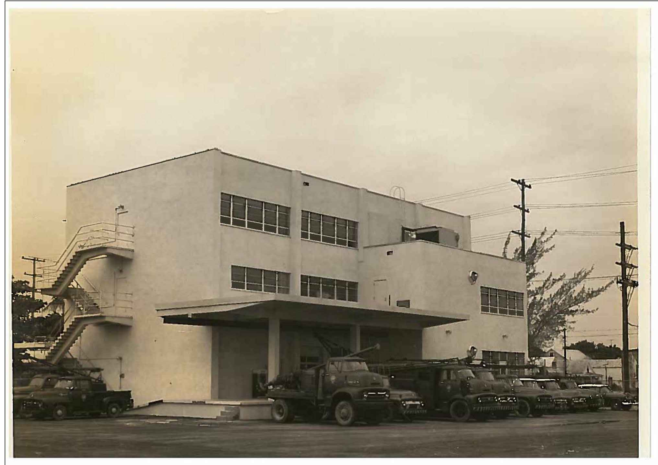
4 HI HISTORIC PHOTOGRAPH OF THE NORTH EXTERIOR ELEVATION BEFORE EAST ADDITION
