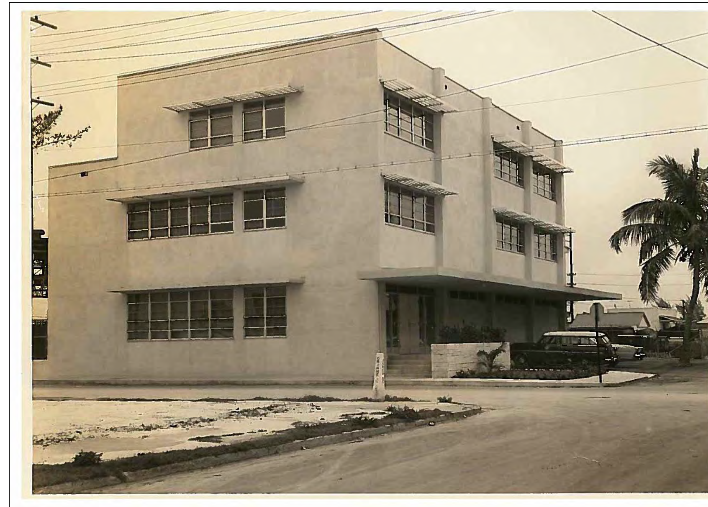
3 HISTORIC PHOTOGRAPH OF THE WEST EXTERIOR ELEVATION BEFORE EAST ADDITION
