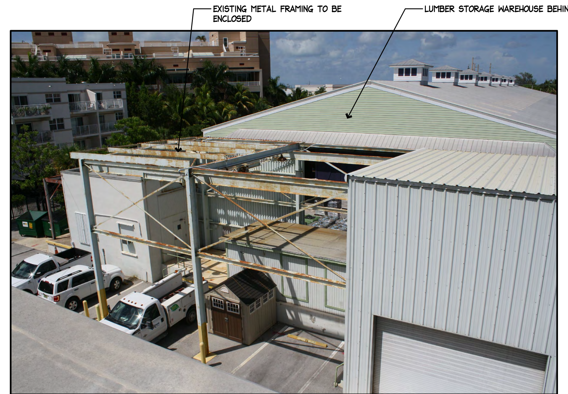
7 PHOTO OF EXISTING STRUCTURE A6.3 N.T.S.
