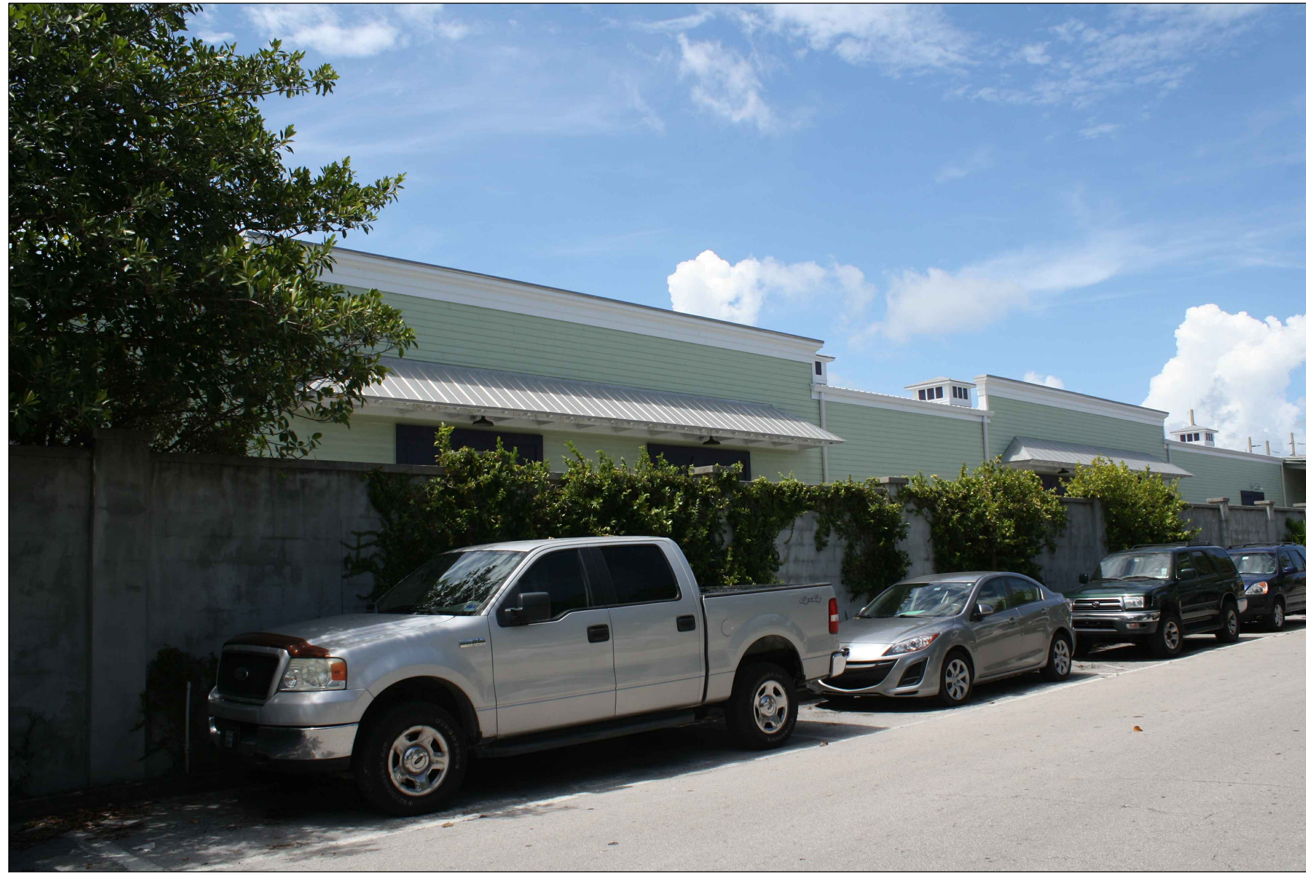
4 H3 STRUNK HARDWARE - NEIGHBOR ON EAST SIDE OF BUILDING
