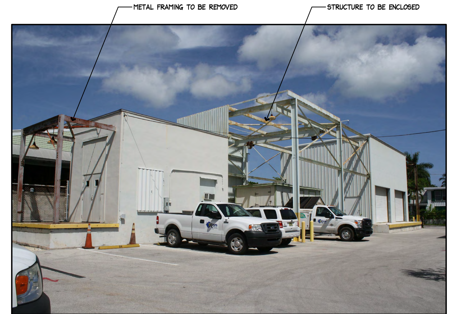
6 PHOTO OF EXISTING STRUCTURE A6.3 N.T.S.
