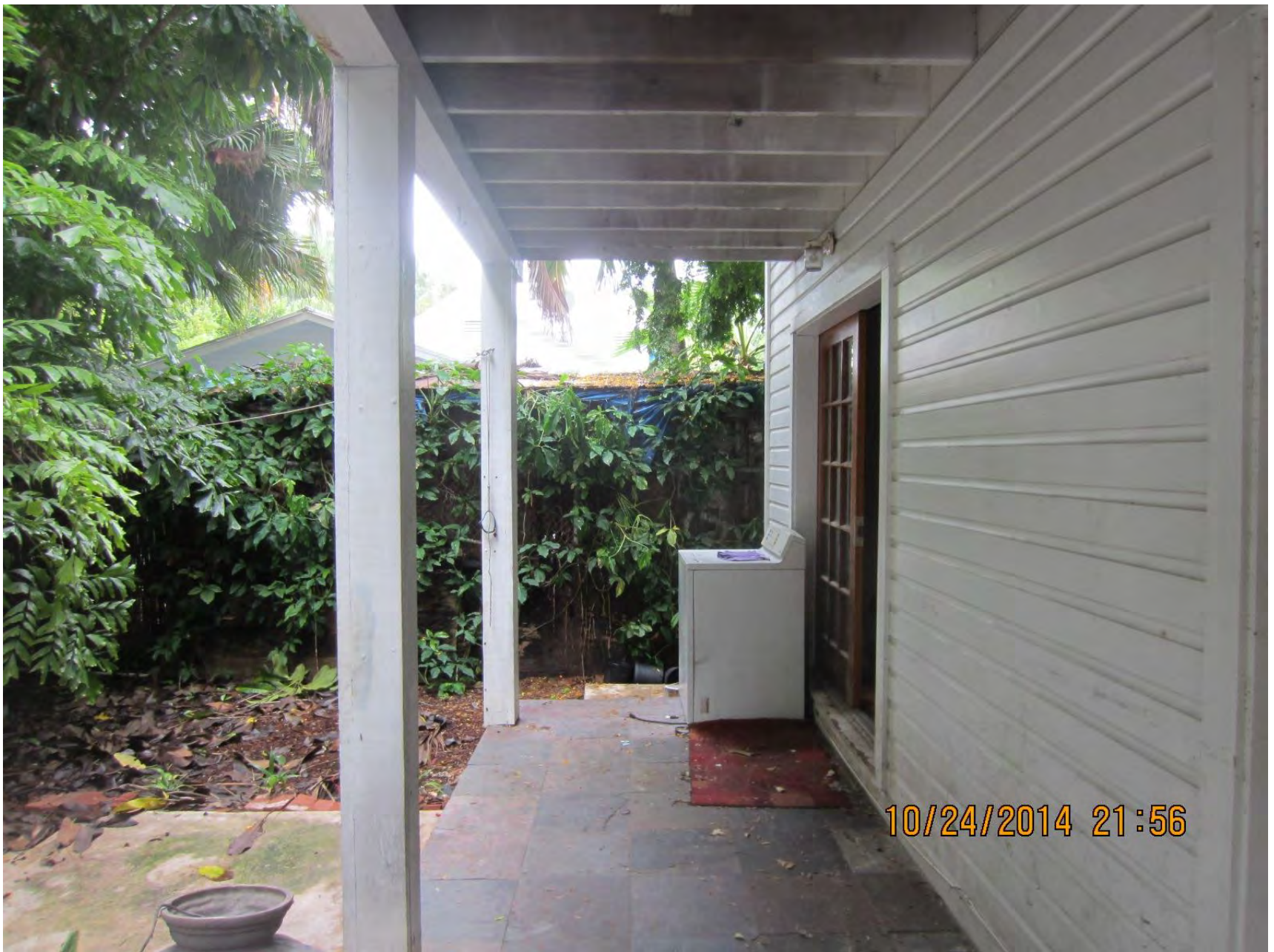
Front porch of existing guesthouse.
