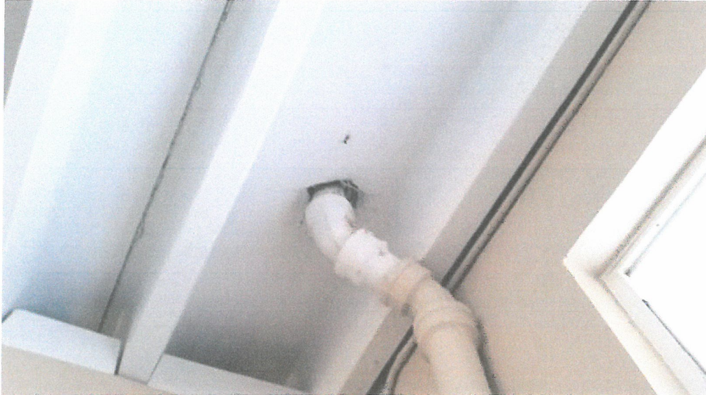
Figure 5. Piping penetration through the slab.
