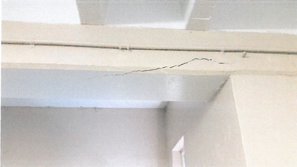
Figure 13. Concrete spalling along the cast-in-place concrete beams. Grade level interior spaces.
