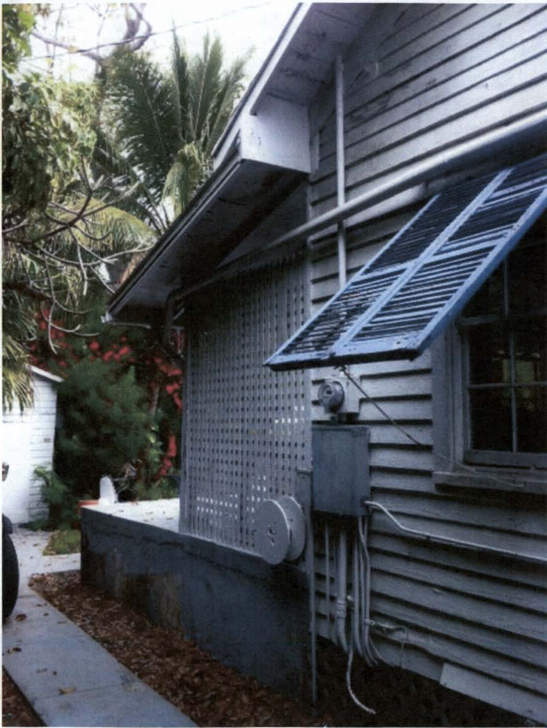
1021 FLEMIING STREET - REAR LEFT SIDE VIEW
