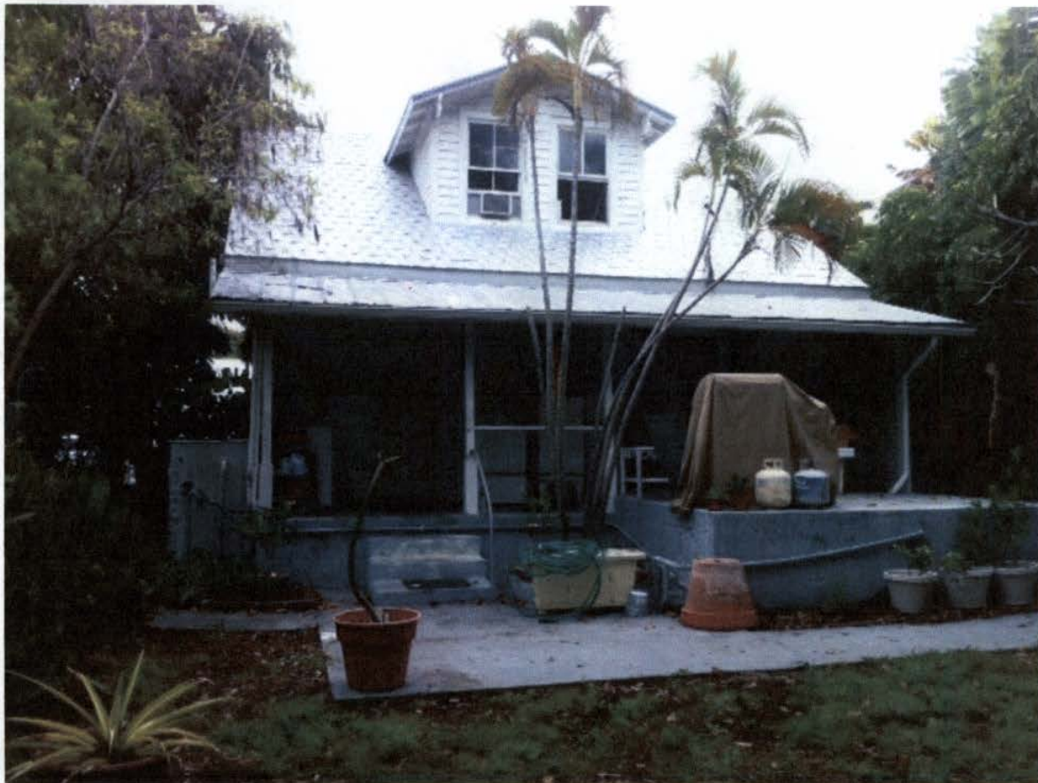
1021 FLEMIING STREET - REAR VIEW
