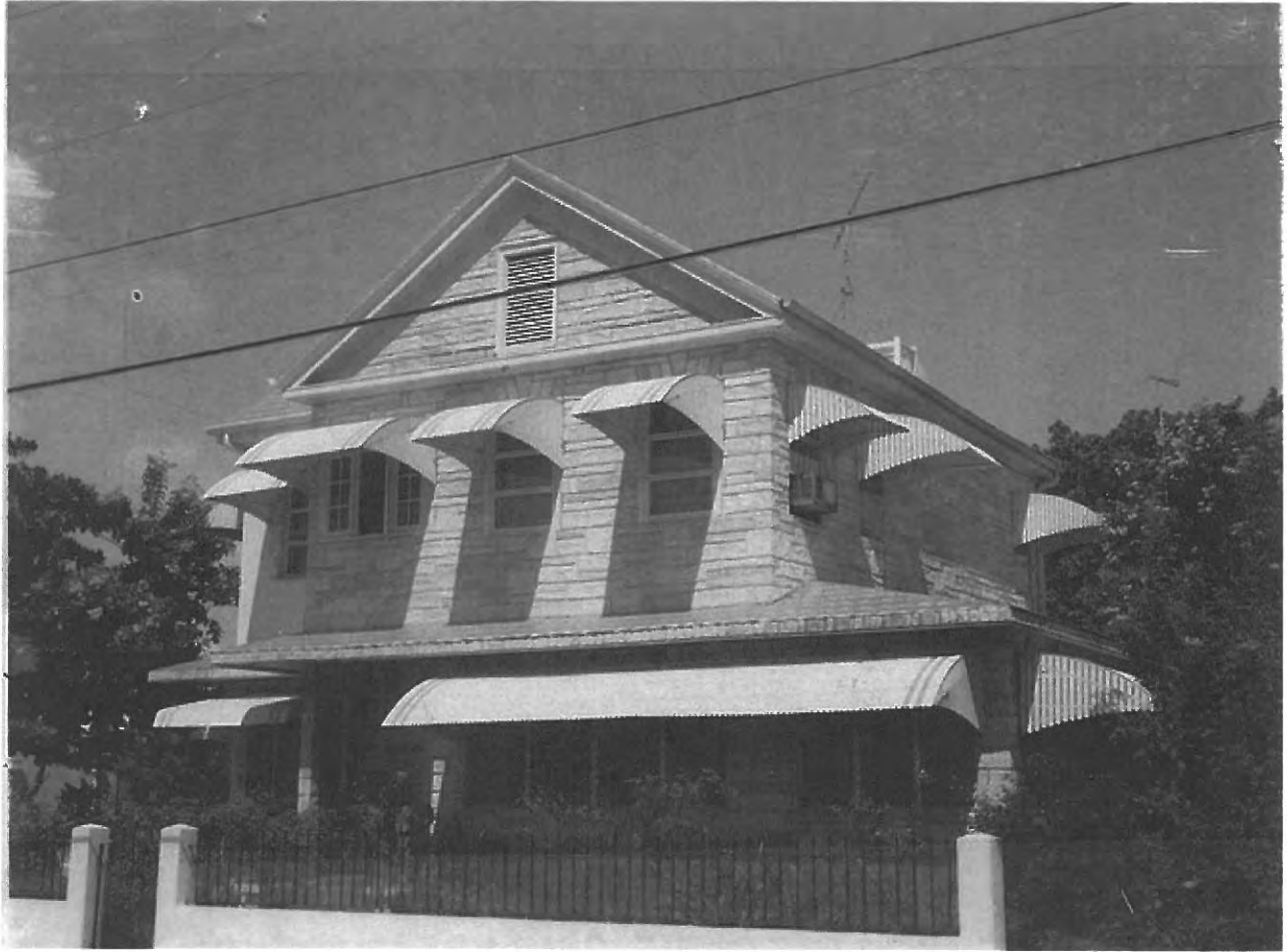
Photo taken by the Property Appraiser's office c1965; 517 Elizabeth St.; built 1953. Monroe County Library
