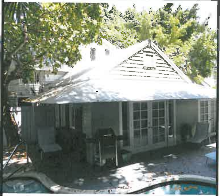
Exterior rear elevation looking at outdoor deck
