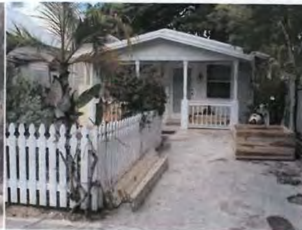
House before recent renovations (2007).
