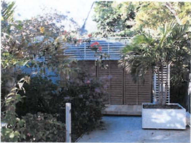
Previous renovation with shutters down.
