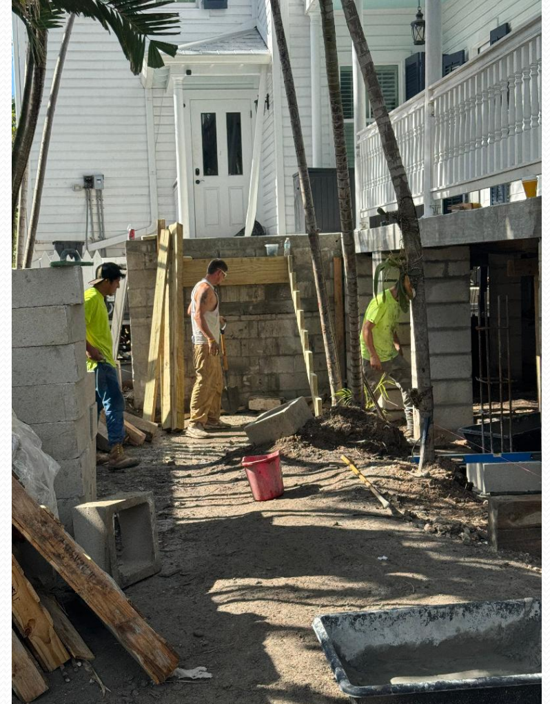
408 United...Done 2000, attached garage to house!
