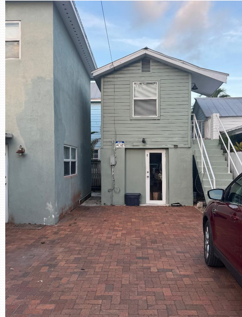
Off of Whitehead Street- extended roof overhang
