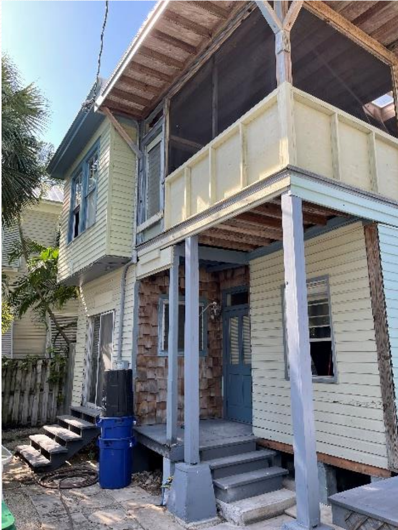
Prior to Lift
