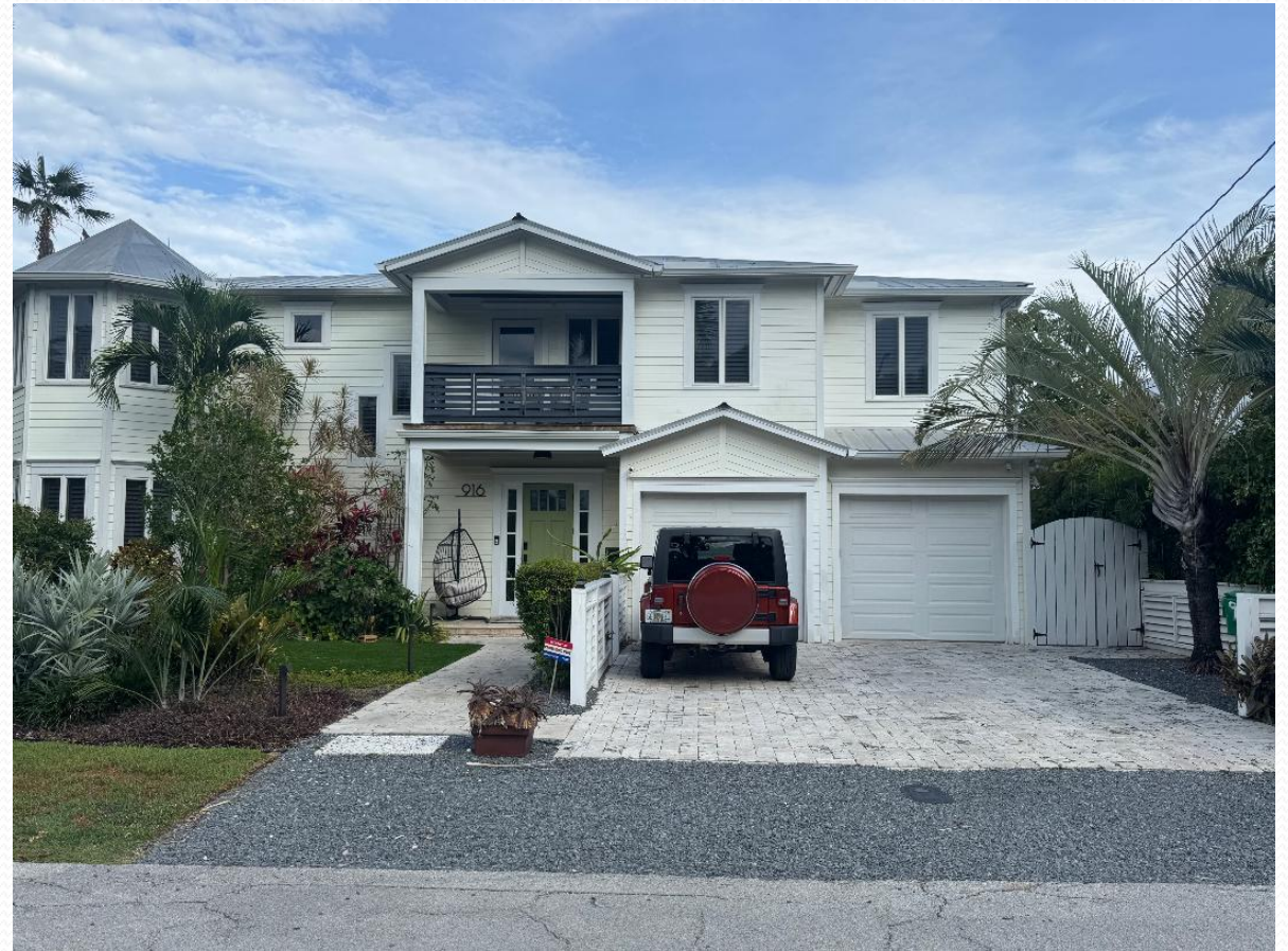
916 Washington Street, Attached to house
