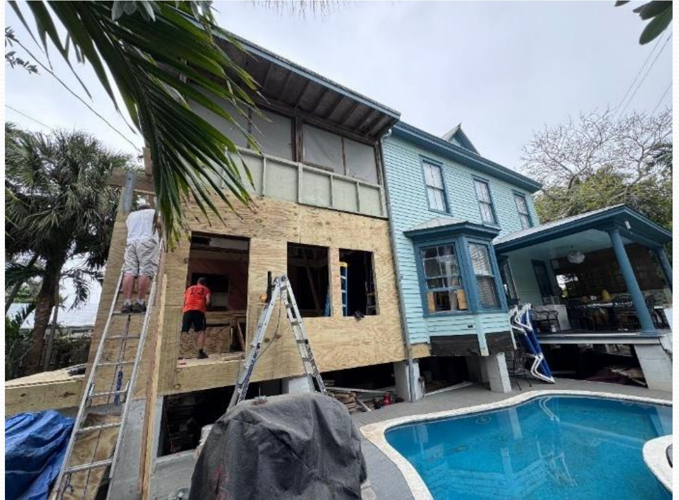
After lift and rebuild of north wall that fell off
