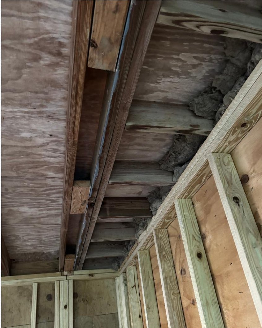
East Joist addition 1975+ Inside
