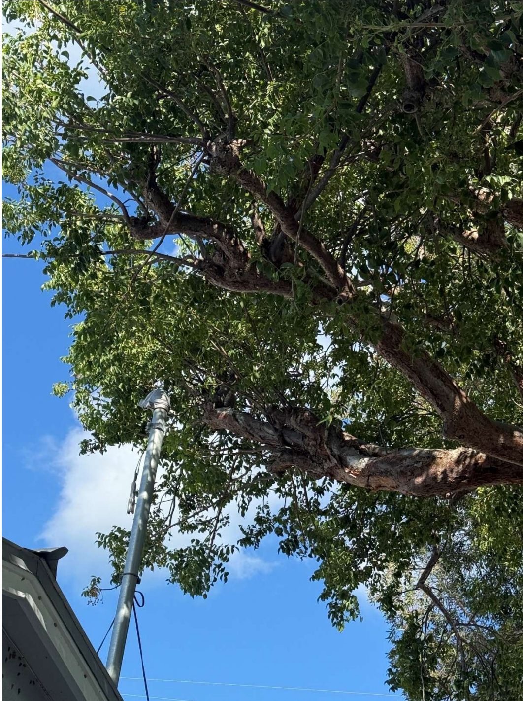
Tree is too close to neighbors electrical service mast.
