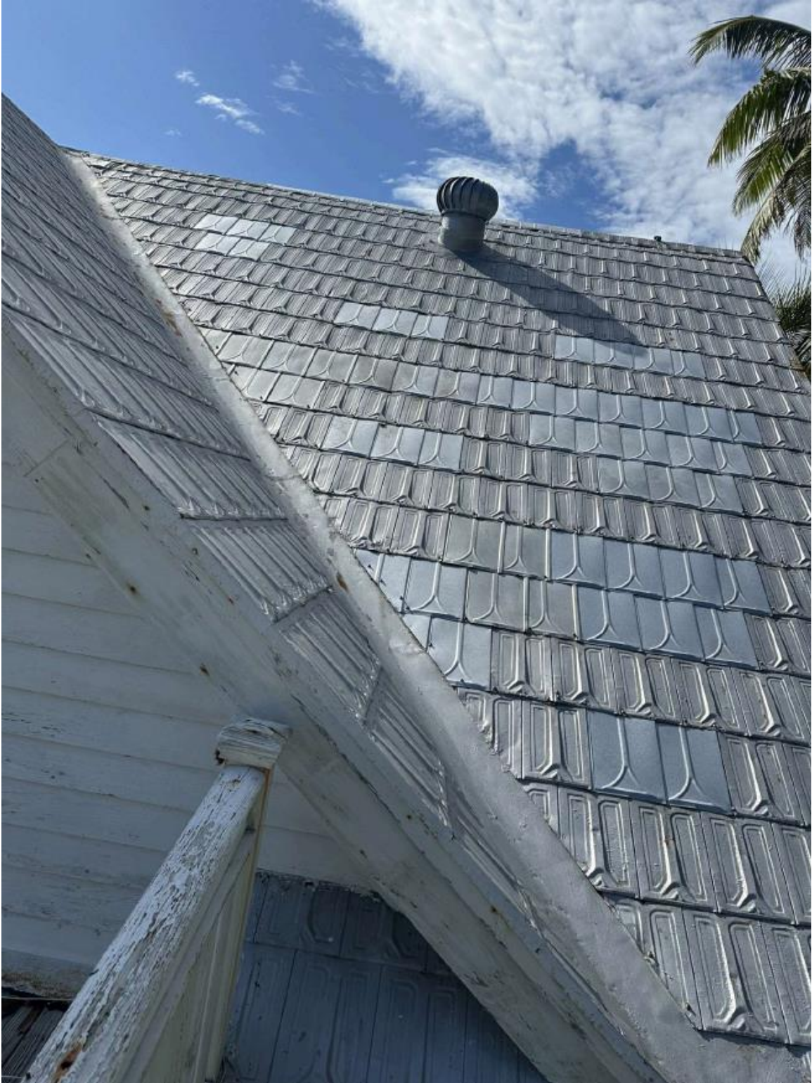
Photo of property under review. Metal shingles in front elevation facing South Street.
